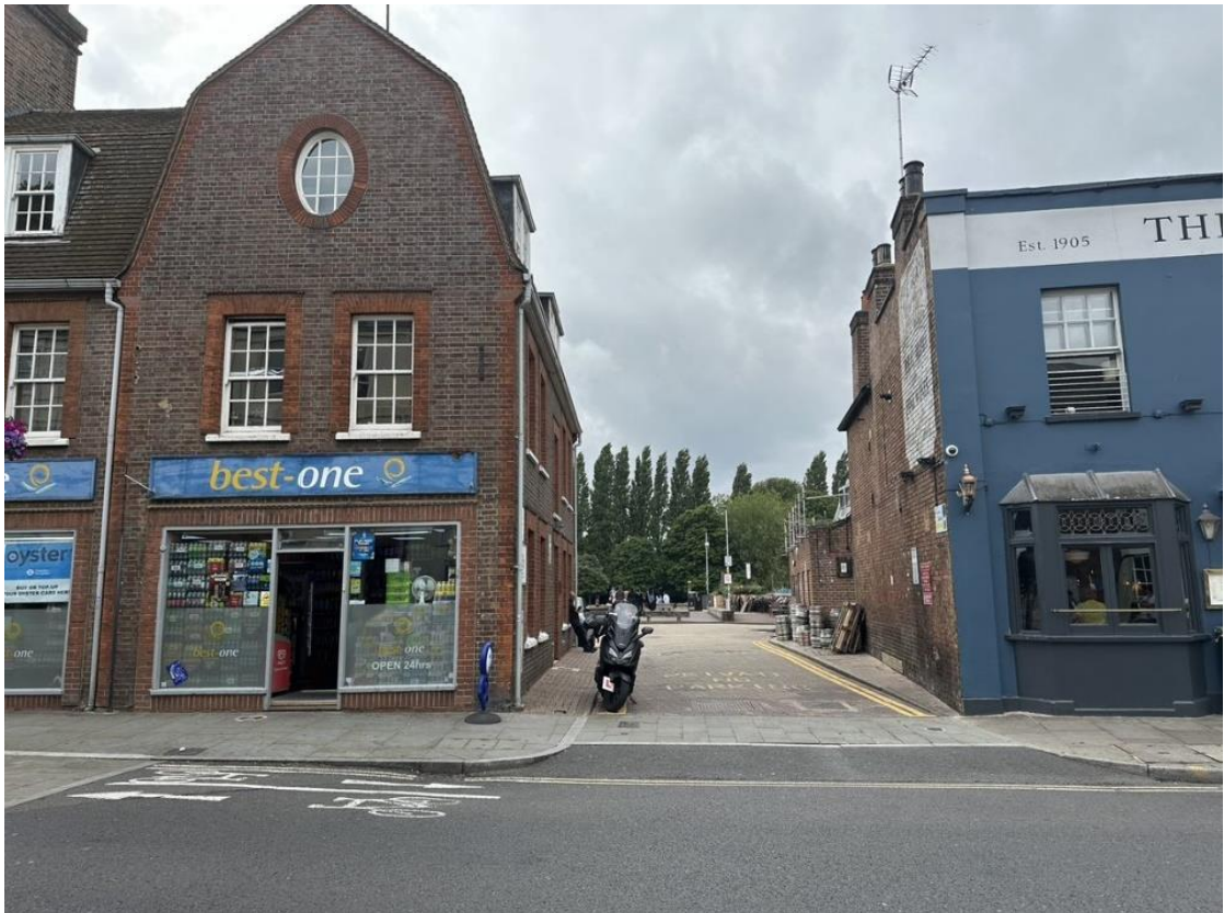
Figure 4.2 The site viewed from High Street through Ram Passage
