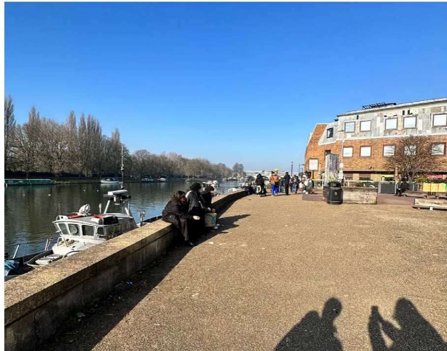
Existing raised river wall
