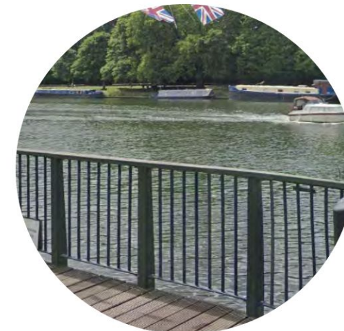
Simple / traditional railing
