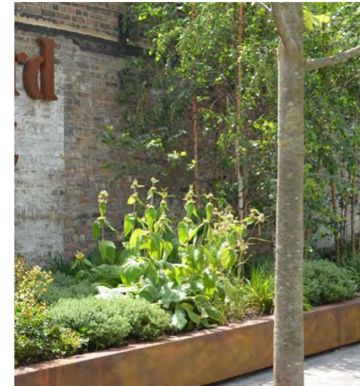
Raised planting beds incorporate powder coated steel edges
