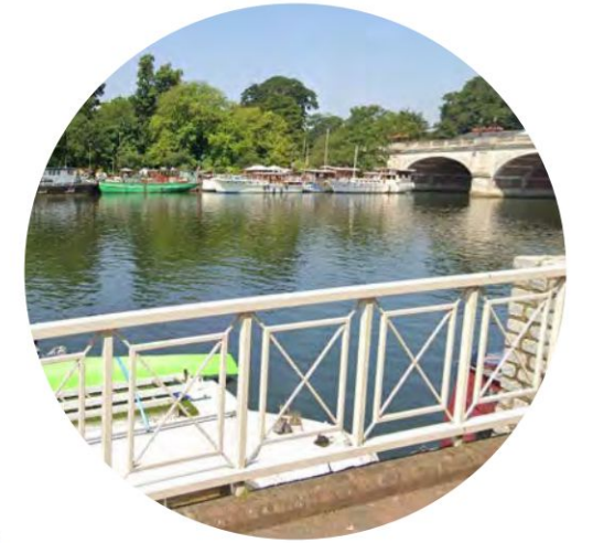
Powder coated metal railing
