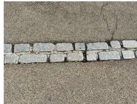
Natural stone setts to be used to demarcate site along the riverfront
