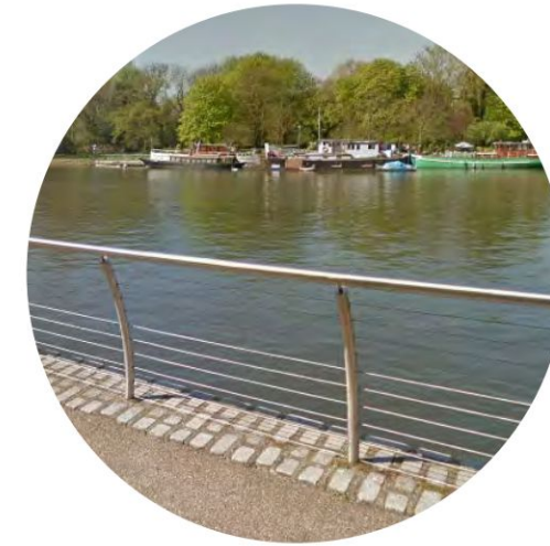
Existing steel and wire railing
