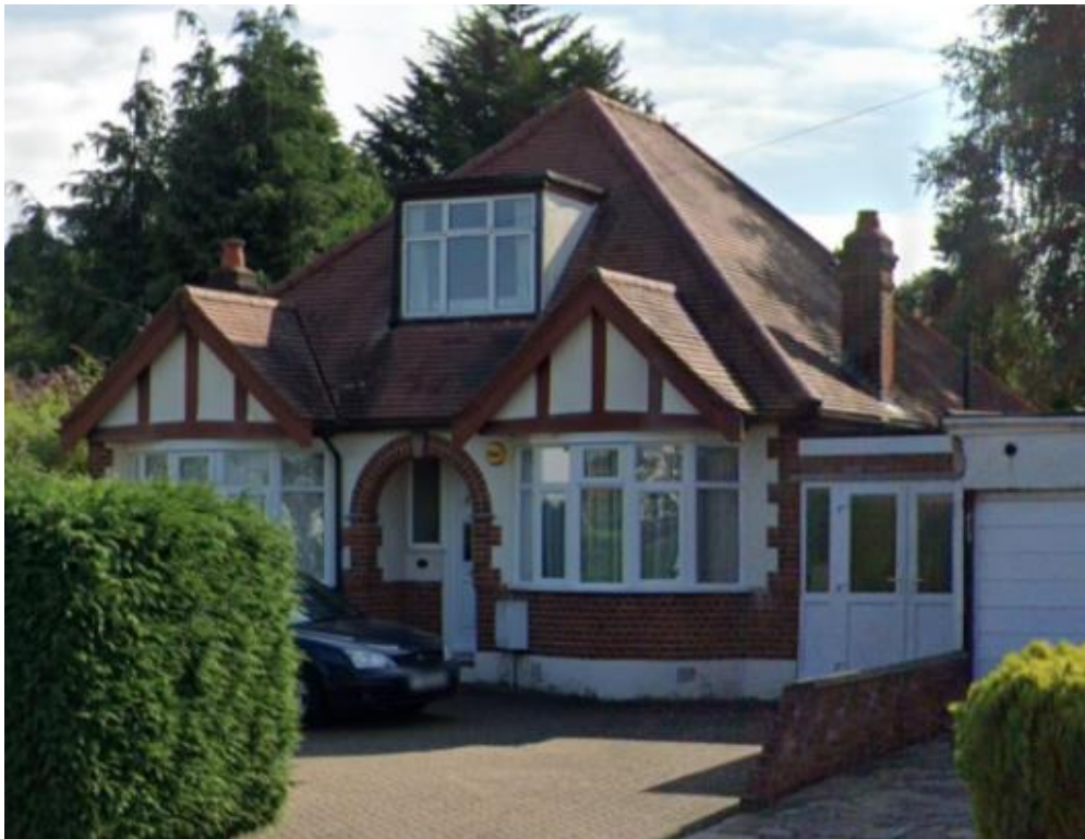
Figure 2: Street View image showing 42 Lyndhurst Avenue
