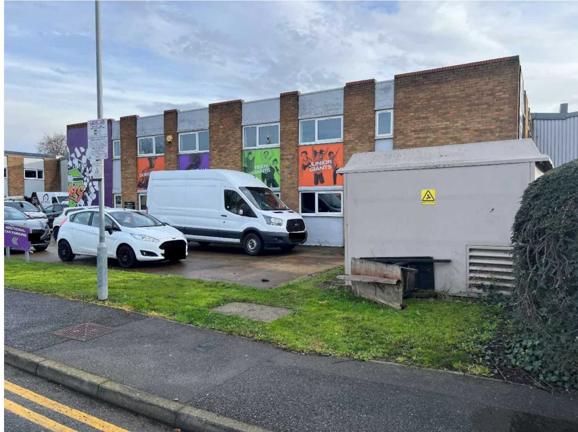
View of existing substation (to be retained) and Unit B3 offices (to be demolished)
