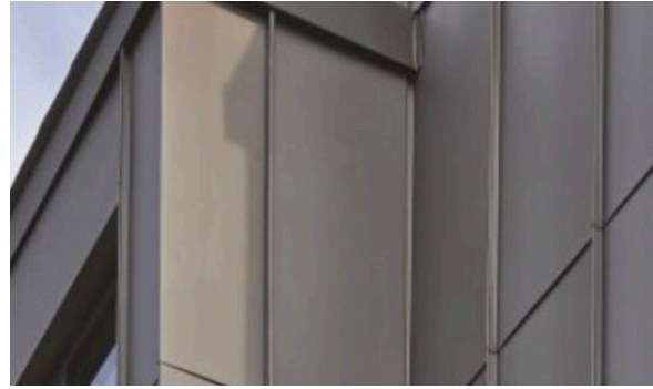
a Metal standing seam zinc roof - VM zinc 'PIGMENTO Grey' with matching rainwater goods
