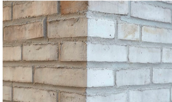
b White brick - Egernsund Tegl 'White Marble' 65mm with CEMEX 'Dove Holes White' premix mortar
