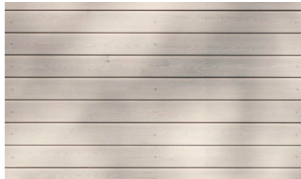
c Timber Cladding - 65mm open joint horizontal Siberian Larch cladding treated with SiOO X 'original'
