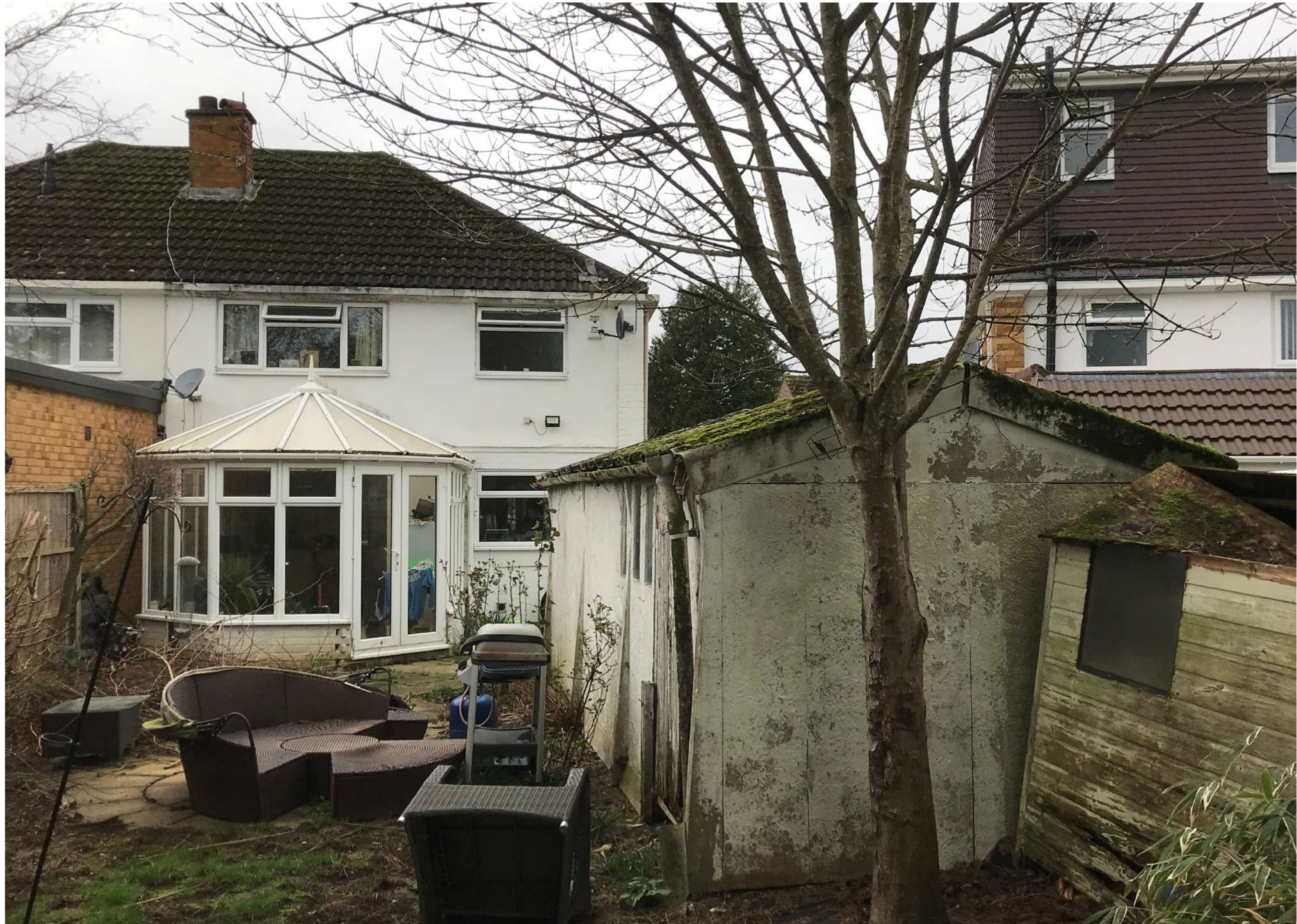
6 Ashbrook Road : Existing Rear - East Elevation : The Conservatory & The Garage are to be demolished:
