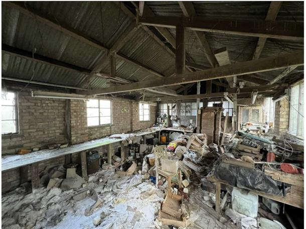
It has a profiled cement board sheet roof cover which is supported by timber purlins in three lines on each pitch.
