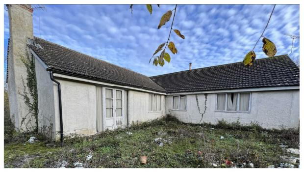
The walls were inspected internally and externally and they are free from any significant cracking. This is a strong indication that the foundations are adequate for the site.
