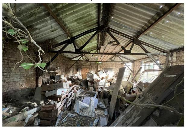
It has a profiled cement board sheet roof cover which is supported by steel angle purlins.
