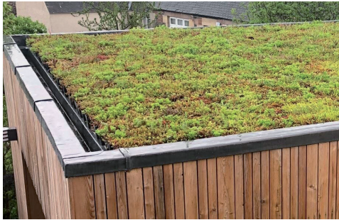
Flat sedum roof
