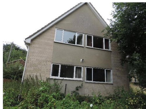
Plate 2: House (B1) Northern Aspect
