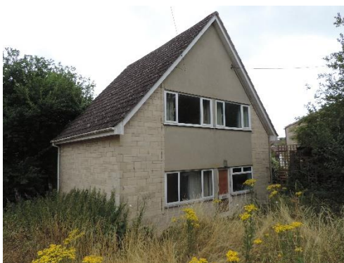
Plate 1: House (B1) Southern Aspect
