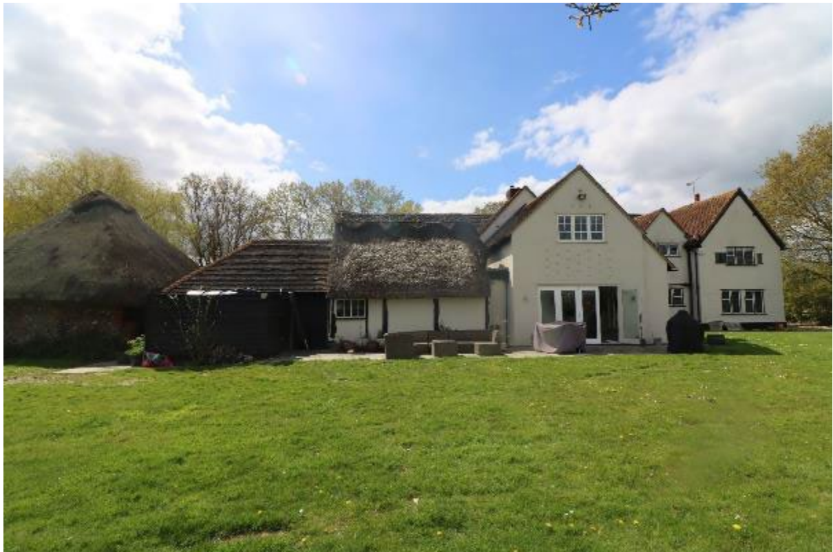
Image 4: Rear Elevation (cement render and pargetting). North-East
