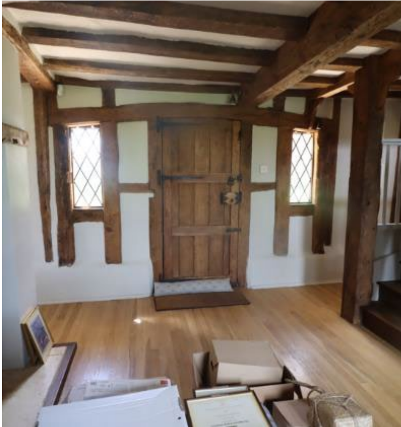
Image 5: Entrance Hall - Example of the concrete and modern floors throughout the ground floor and the cement to the interior plinth and gypsum on the internal walls- all done during the 1970s.
