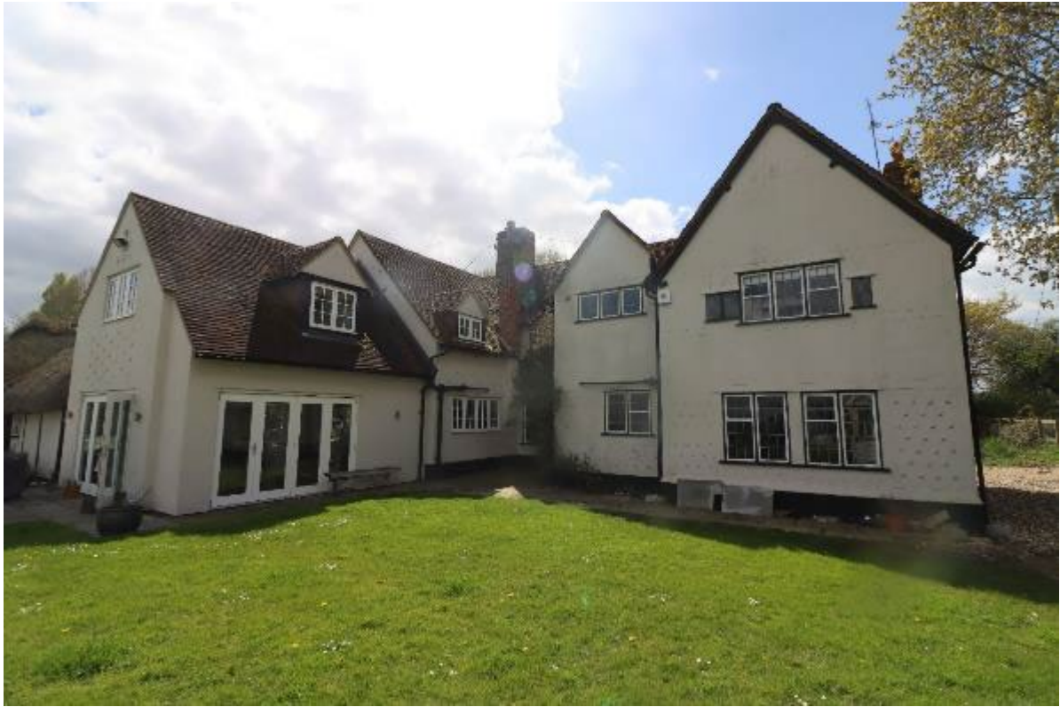
Image 3: Rear elevation (cement render). North-West
