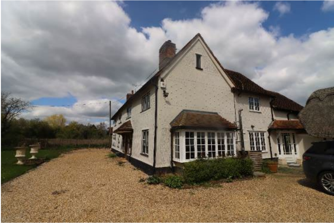
Image 1: Front/side elevation (cement render). South-East.
