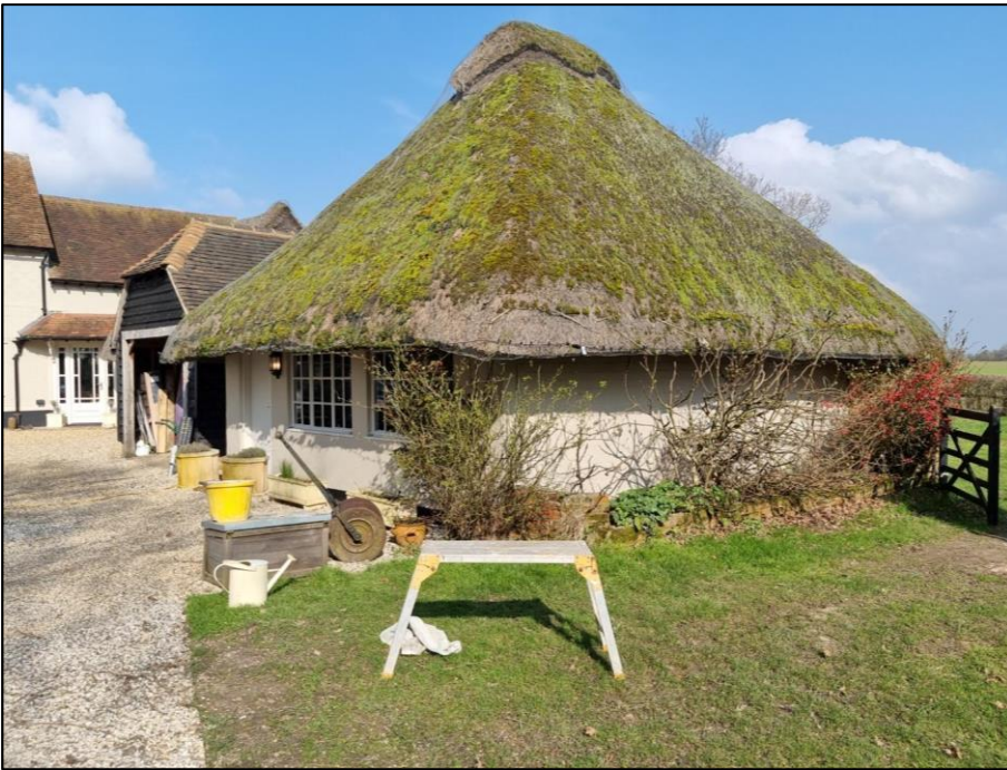
Thatched gym building. Viewed from the southeastern corner.
