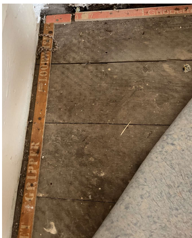
C20 MACHINE CUT TIMBER FLOORBOARDS TO LOWER SITTING ROOM FLOOR
