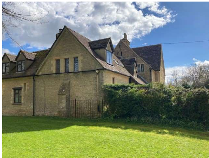
This shows the northern elevation of The Forge looking at it from the Village Green
