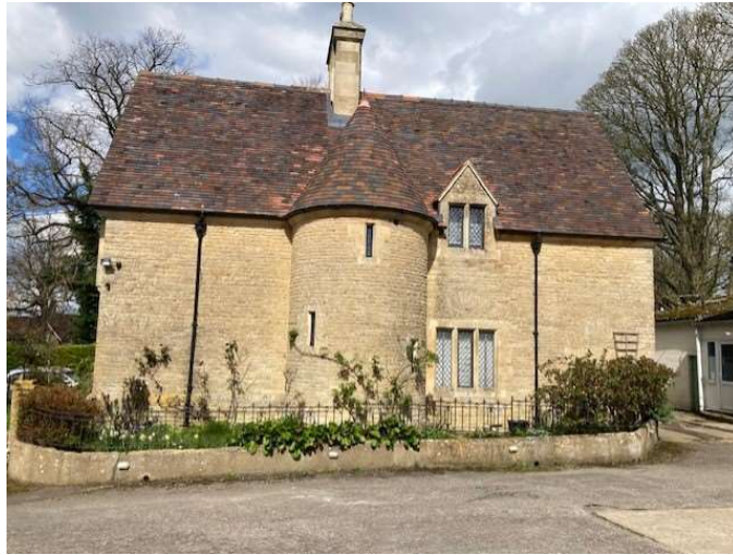
The above shows the southern elevation of the Forge from the Forge MOT Garage car park
