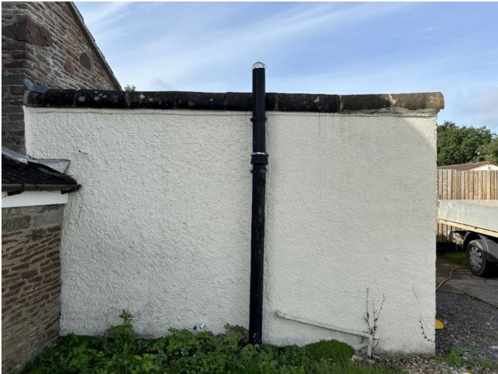
Photograph 5: B1, eastern elevation
