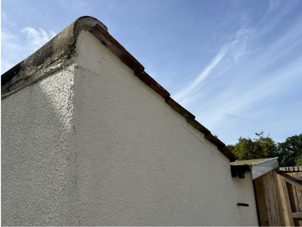
Photograph 20: B1, 'eave' of northern elevation
