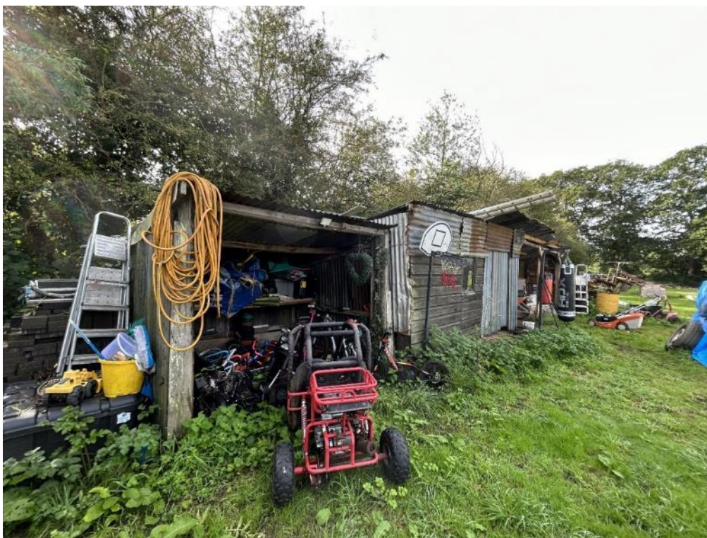
Photograph 7: B2, eastern and southern elevations
