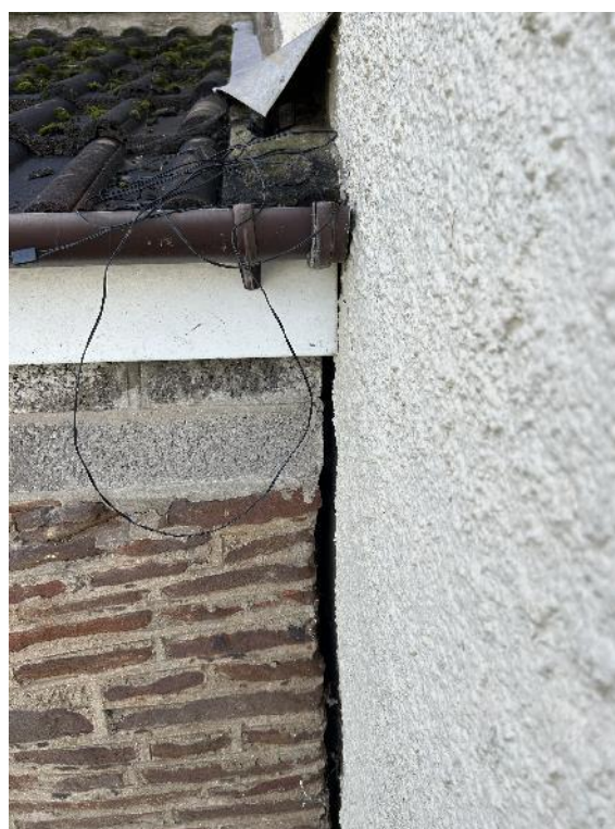
Photograph 23: B1, connection point to retained building, no evidence of bats
