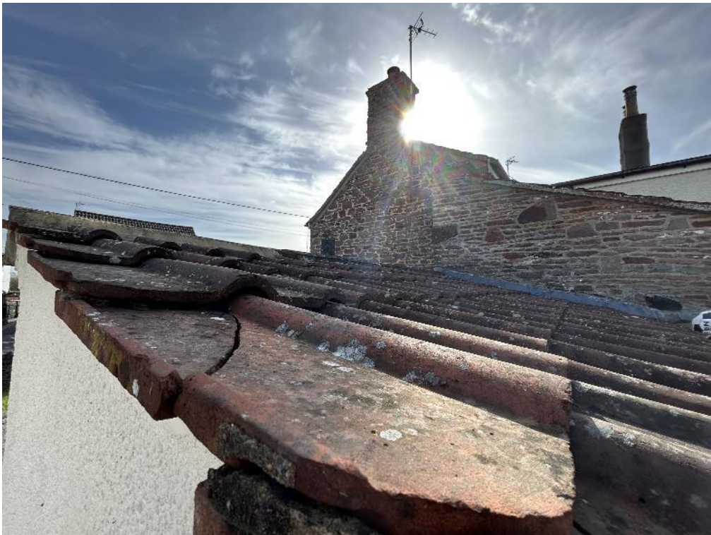
Photograph 21: B1, ridge line and tiling of roof
