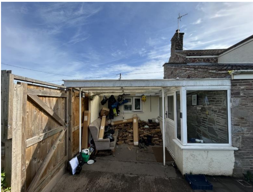
Photograph 6: B1, western elevation
