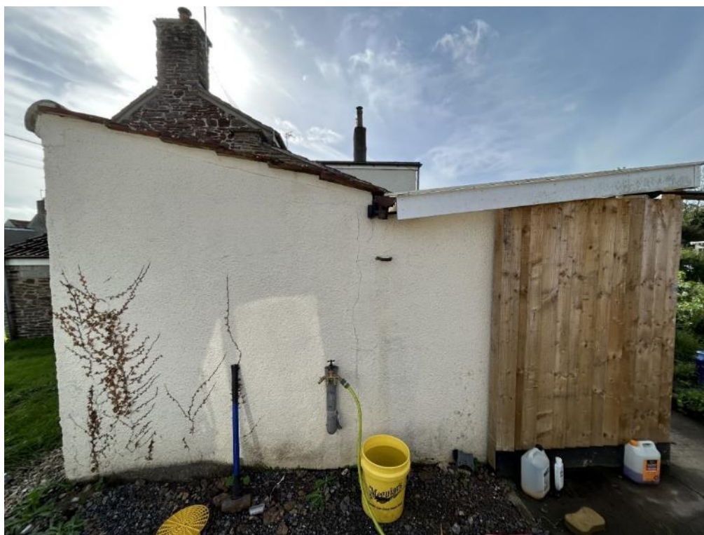
Photograph 3: B1, northern elevation
