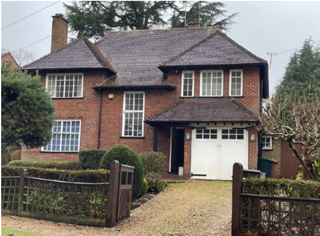
Fig.3: East elevation, including garage with extant permission to be converted to a living space and replaced by a window. The side projection and its small window are seen to the right.
