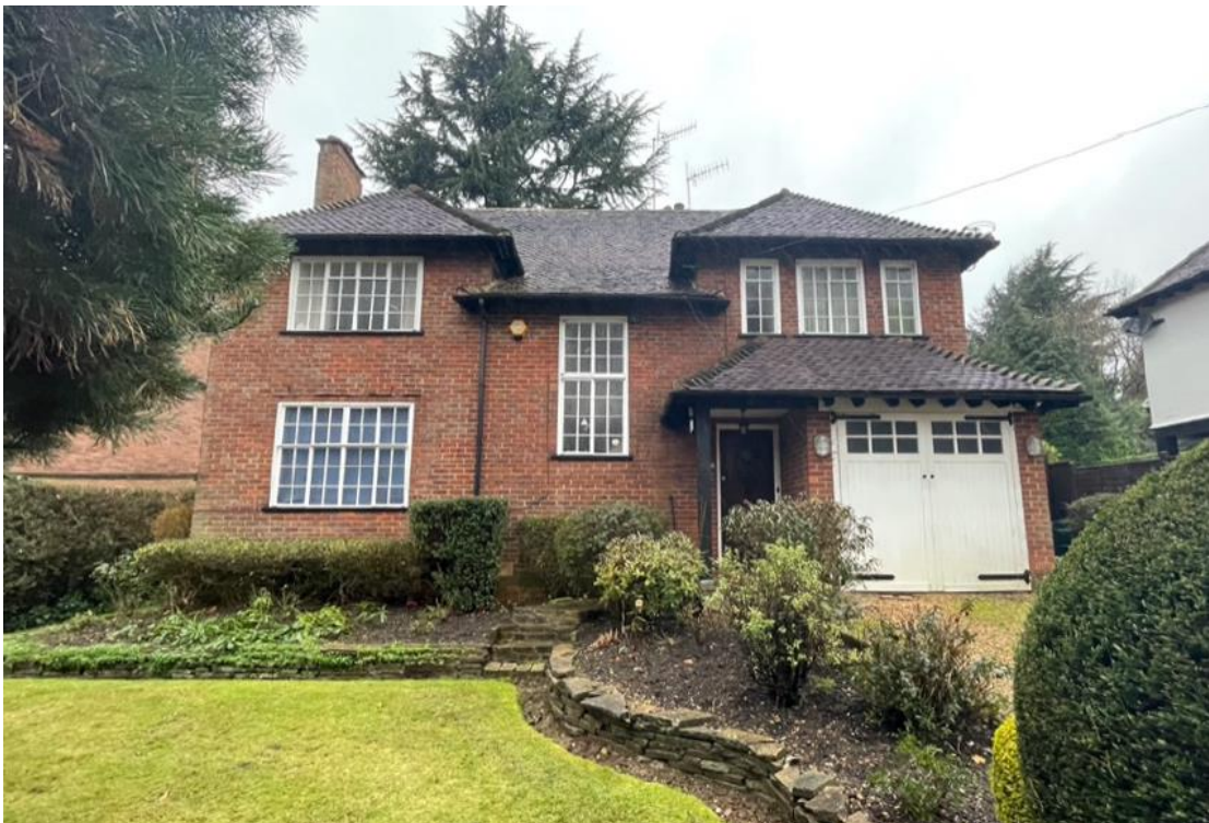
Fig.4: East elevation seen from the front garden.
