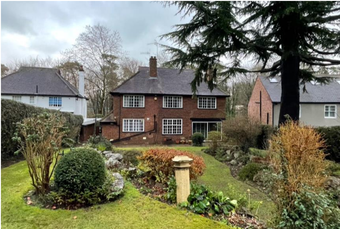
Fig.5: The rear (west) elevation of the property, with modern patio door to right and side projection to the left.
