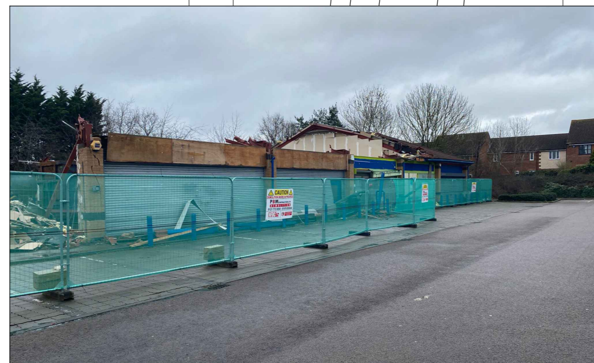
Example image: Double clipped herras panels for demolition works
