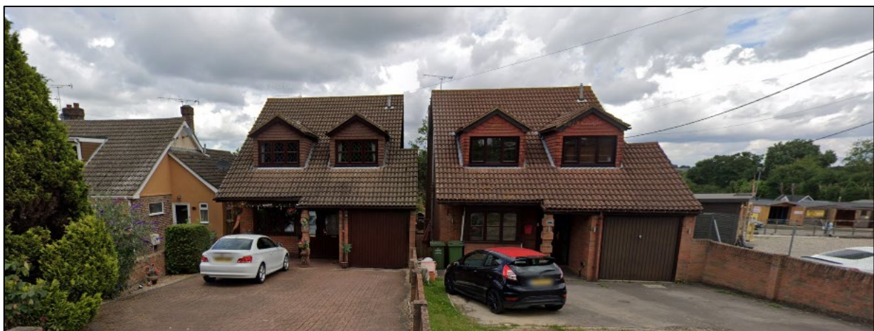
Figure 7: 248-250 London Road, Wickford
