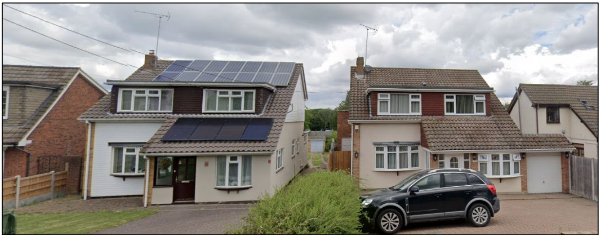
Figure 9: 256-258 London Road, Wickford
