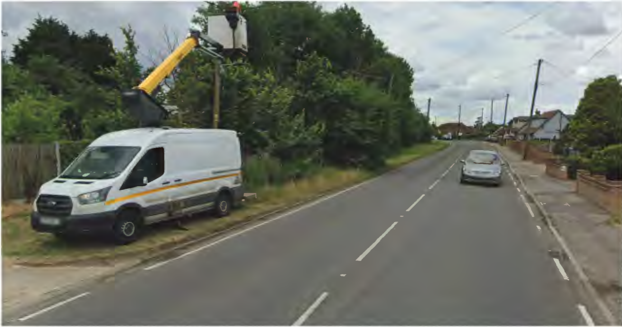
Fig 8. View from site from the East along London Road
