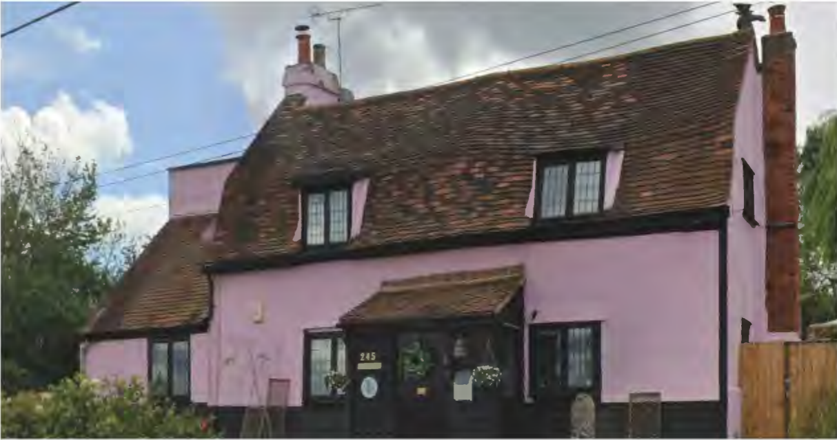
Fig 12. Neighbouring property at 245 London Road
