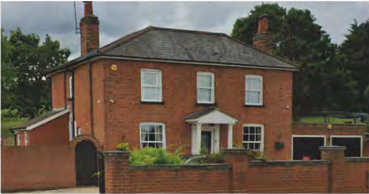
Fig 7. Brick House Farm House
