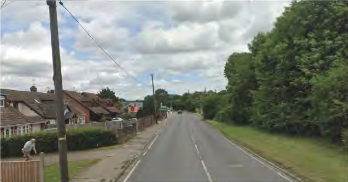
Fig 11. View of site to the right looking east along London Road
