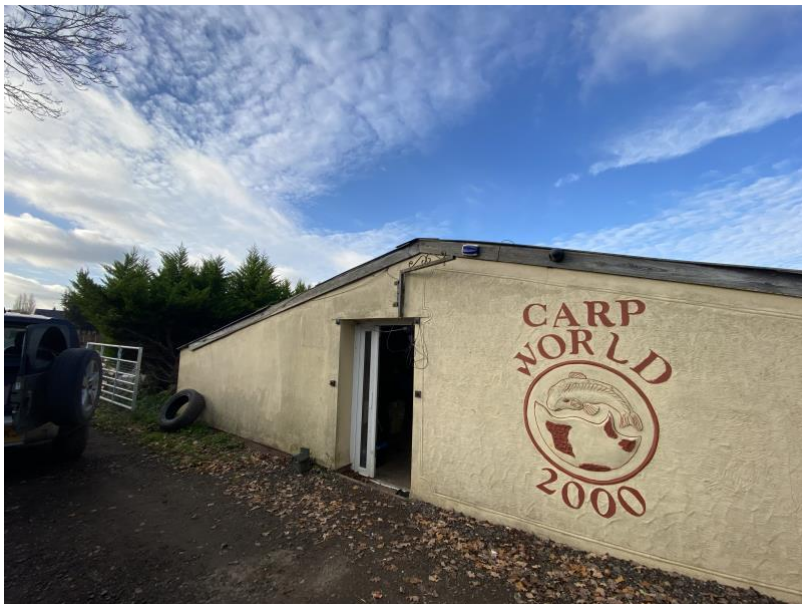
Building B2 exterior.
