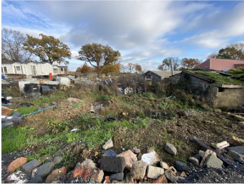
Area of nettle and rubble to the north of the site.
