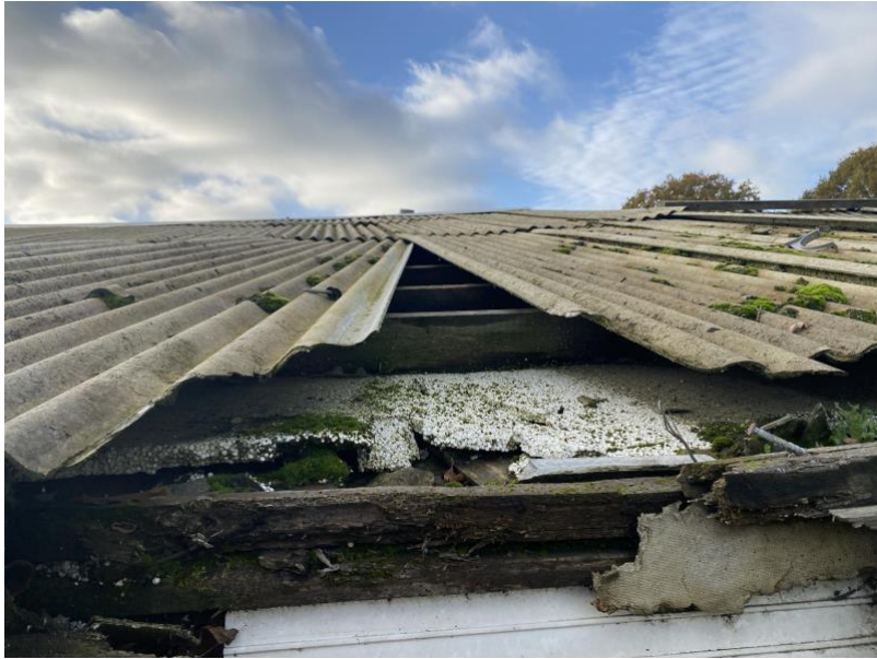
Access points within roof materials on Building B1.
