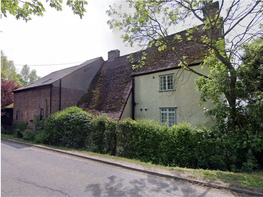
Fig. North Bound View
