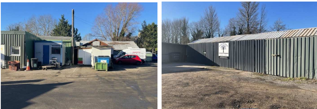
Fig. Existing Units to Rear of Fieldgate Farmhouse
