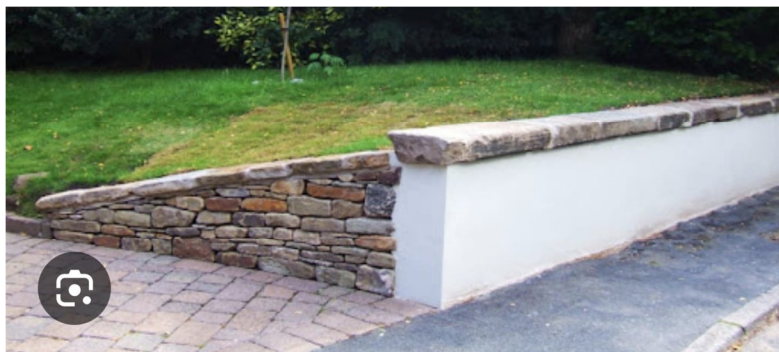
Proposed Driveway Boundary Wall Treatment (Installed at Position A).
