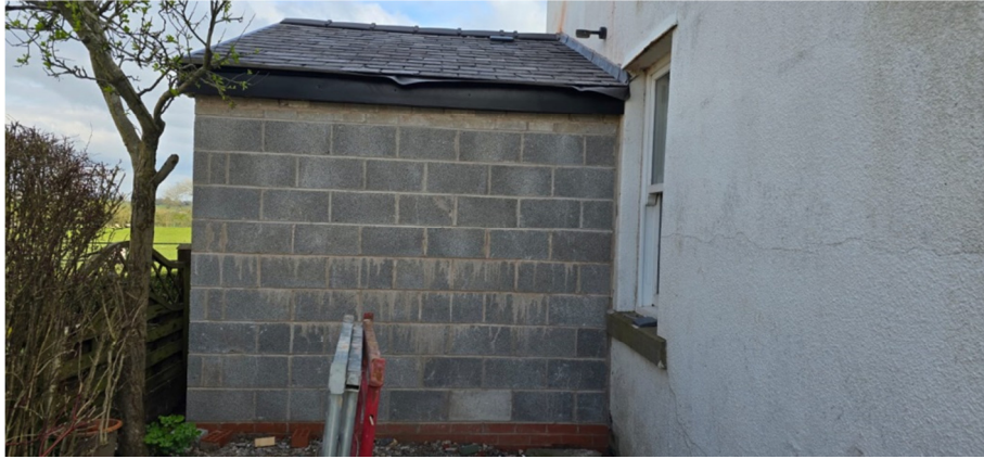
External Side Outbuilding viewed from front AS IS.
