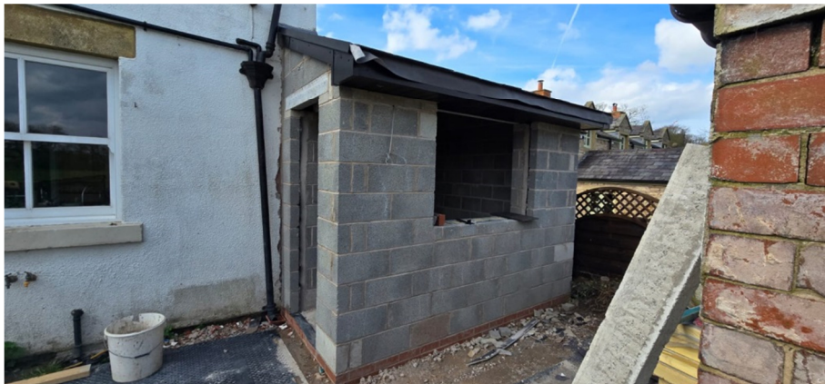
External Outbuilding viewed from Rear AS IS.
