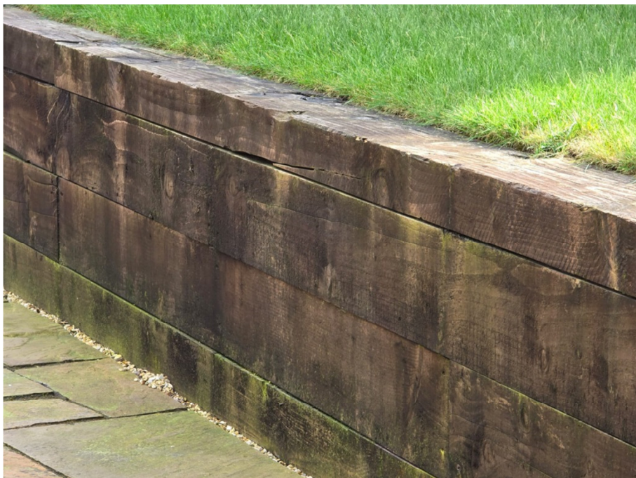
PROPOSED SLEEPER WALLS TO SIDE AND REAR BOUNDARY FENCE. (TO BE INSTALLED AT POSITION B with new Lattice fence over).
