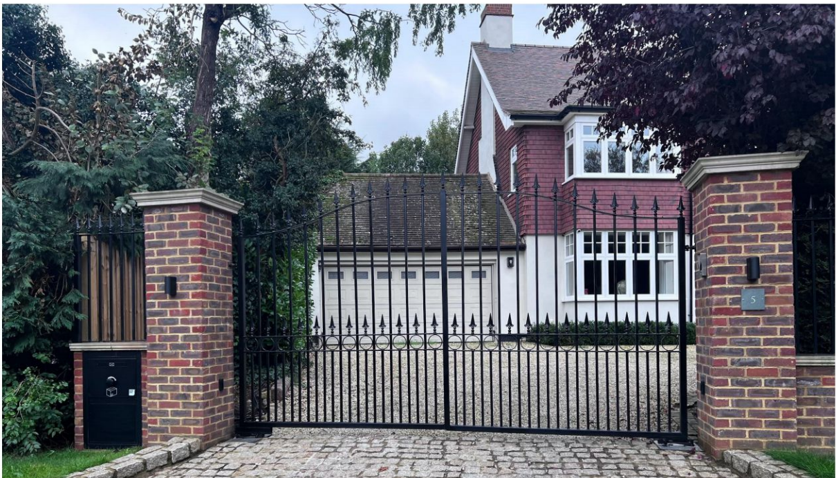
Iron gates, fencing and brick pillars - 5 The Headway
