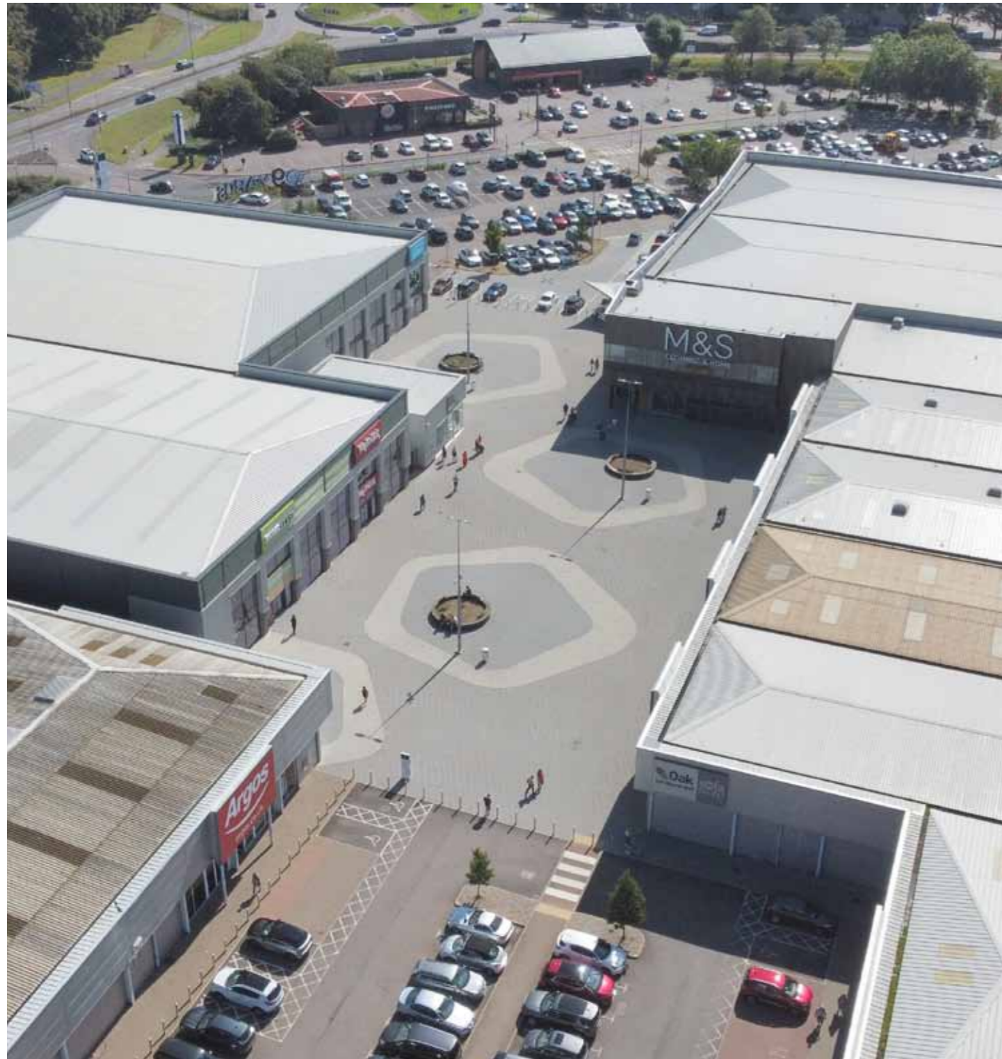
The existing site looking south
