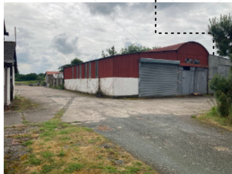
Main Storage Unit 01
