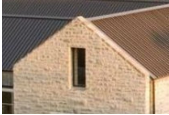
1. Parapet gable wall detail
