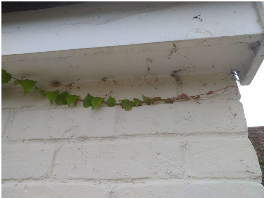
Tight seal between soffit and brickwork on porch
