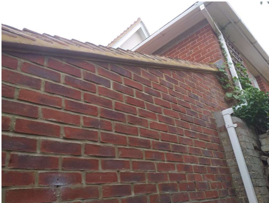
Tight seal between wall and tiles on south eastern corner
