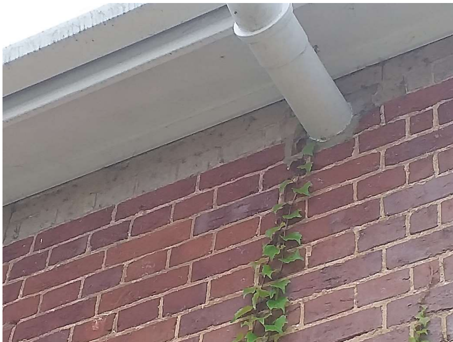
Tight seal between brickwork and soffit
