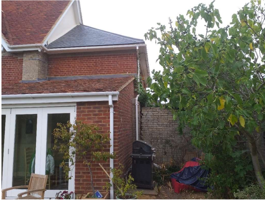
South eastern side of eastern wing
