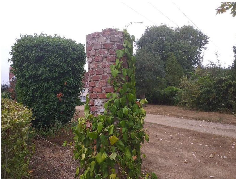
Brick pillars to be removed
