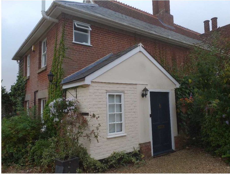
Small porch on northern elevation of eastern wing
