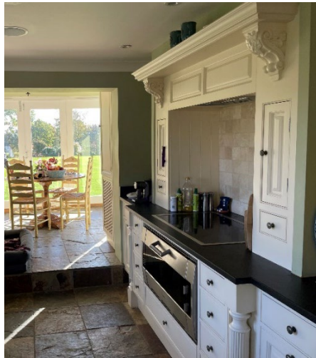
Figure 21. Existing kitchen with C20 lean-to to the south and visible change in floor level which shall be lowered as part of remodelling.
