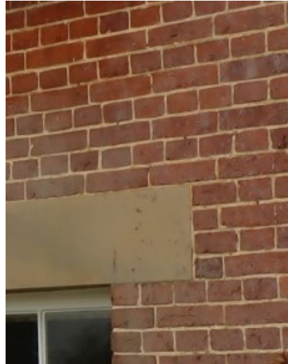
Figure 6. & 7. Red bricks to the external elevations in English Bond with stone details in a york stone or similar to match the existing 4 brick high lintels. The plinth shall be gault bricks to match the existing Hall.
