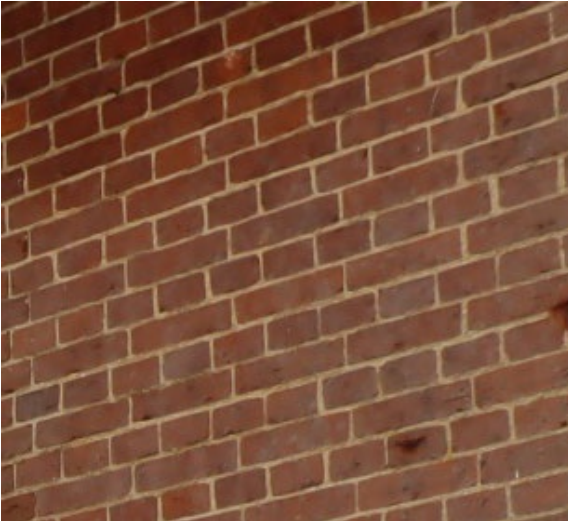
Figure 6. & 7. Red bricks to the external elevations in English Bond with stone details in a york stone or similar to match the existing 4 brick high lintels. The plinth shall be gault bricks to match the existing Hall.
