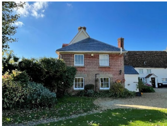
Figure 16. North East (Side) Elevation c.1900 service accommodatin with slate hipped roof.
