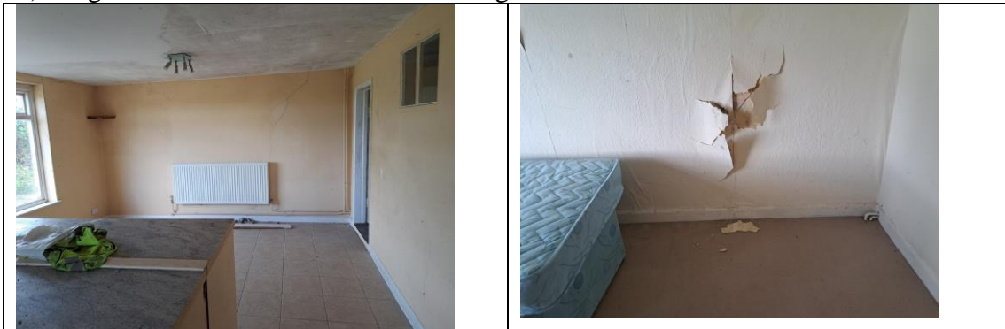
d) Diagonal crack in external wall at both ground floor & 1 st floor level.
