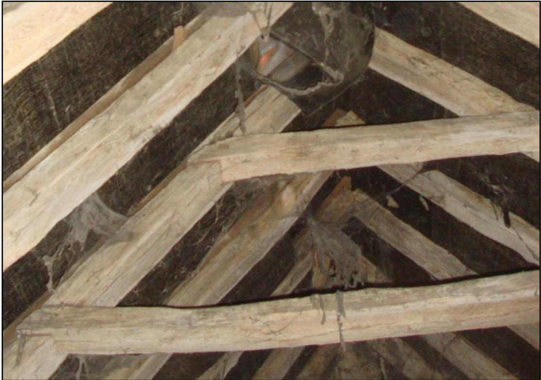
Fig.18 Collar-rafter roof above mid-fifteenth century bay
