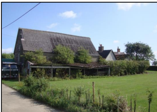
Fig.27 Farm premises (from SW)
