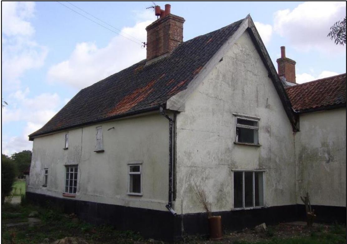
Fig.16 Principal range (south and west elevations)
