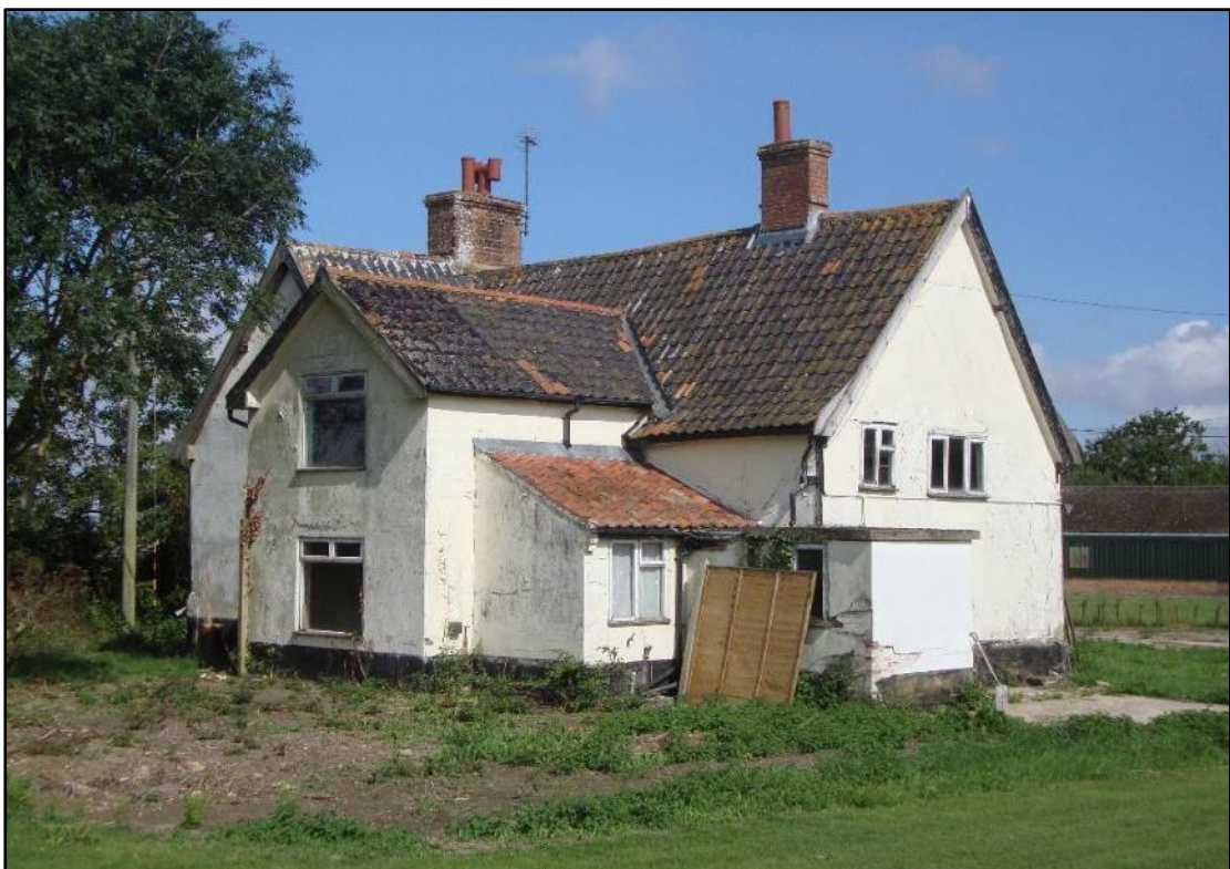
Fig.23 Secondary range (south and east elevations)
