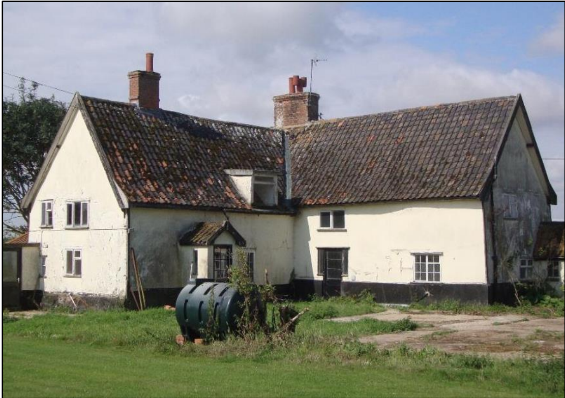
Fig.22 Secondary range (north and east elevations)
