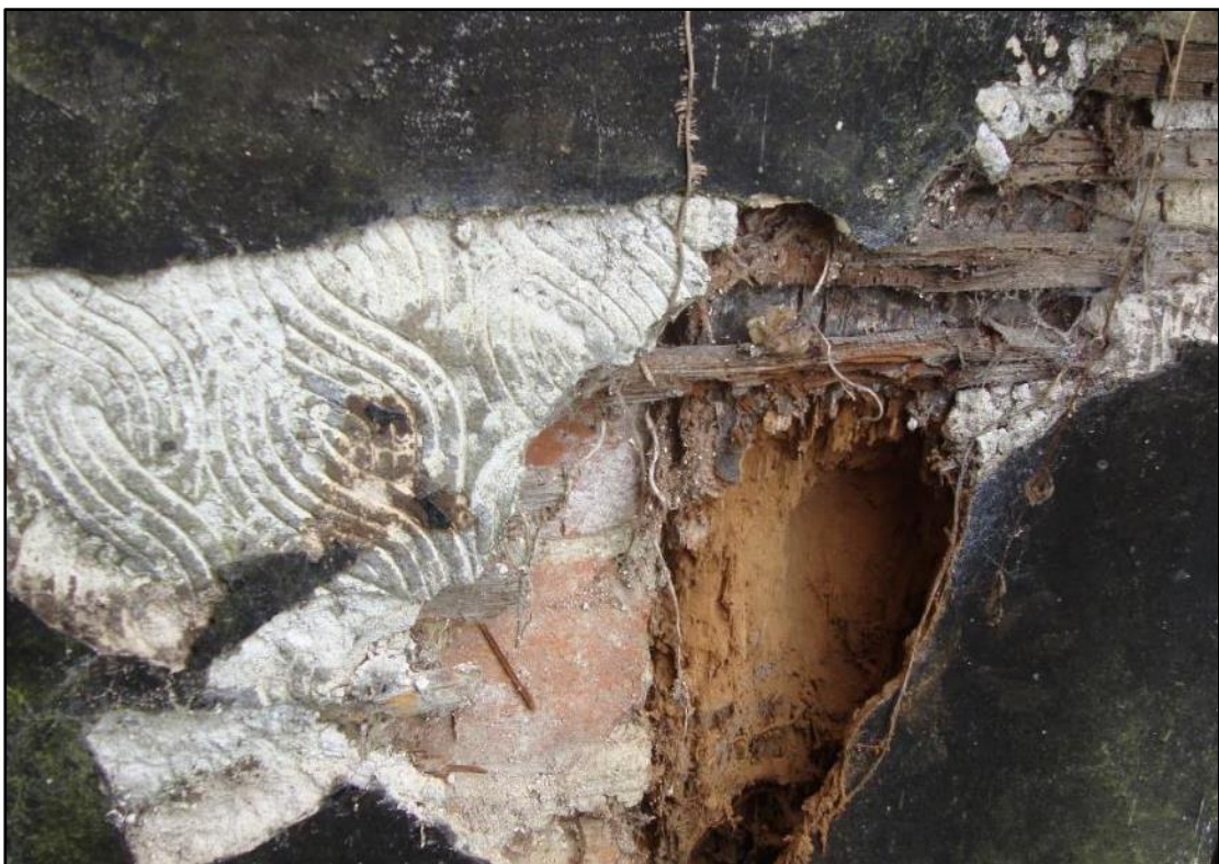
Fig.36 Remnant of incised pargeing on rear service range
