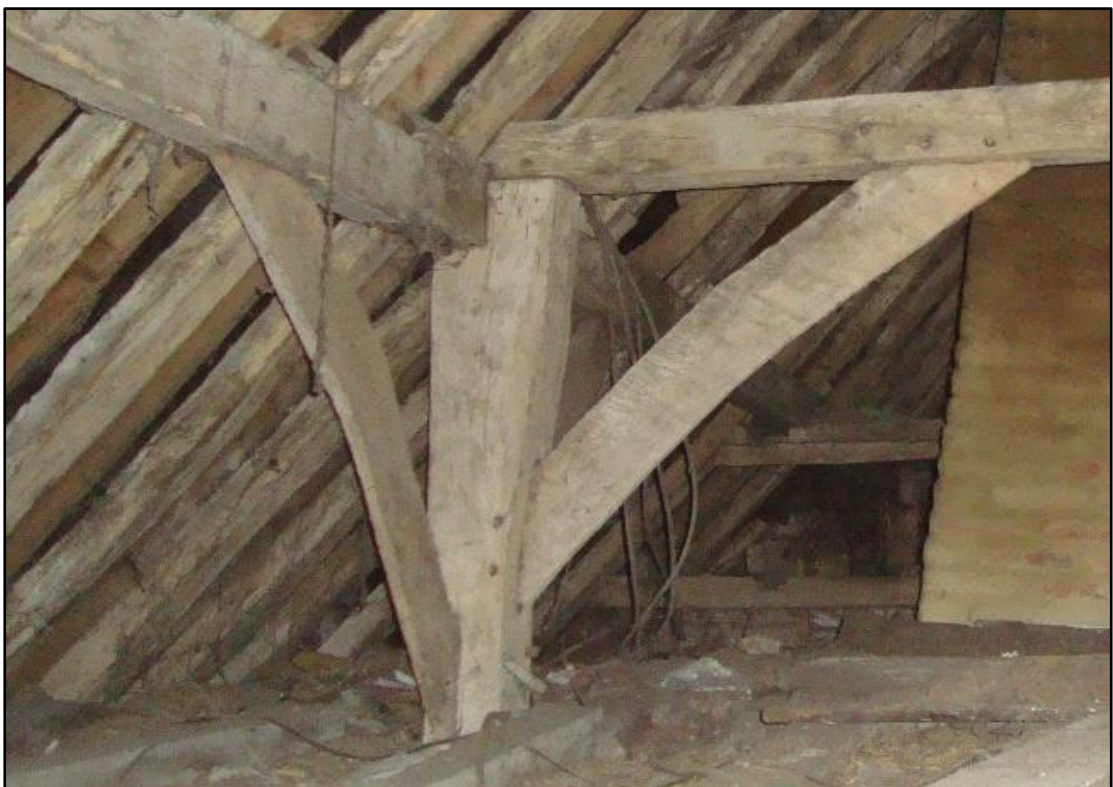
Fig.21 Jowled queen post clasp square-set side purlin
