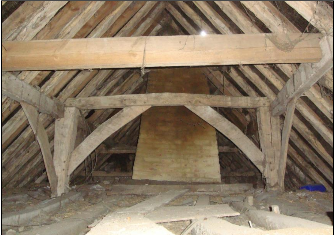
Fig.20 East Anglian queen-post roof above late sixteenth century addition
