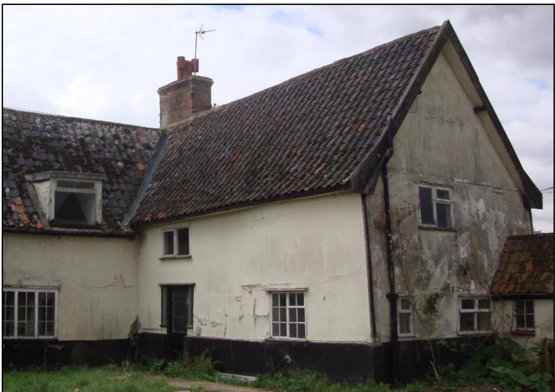
Fig.17 Principal range (north and east elevations)
