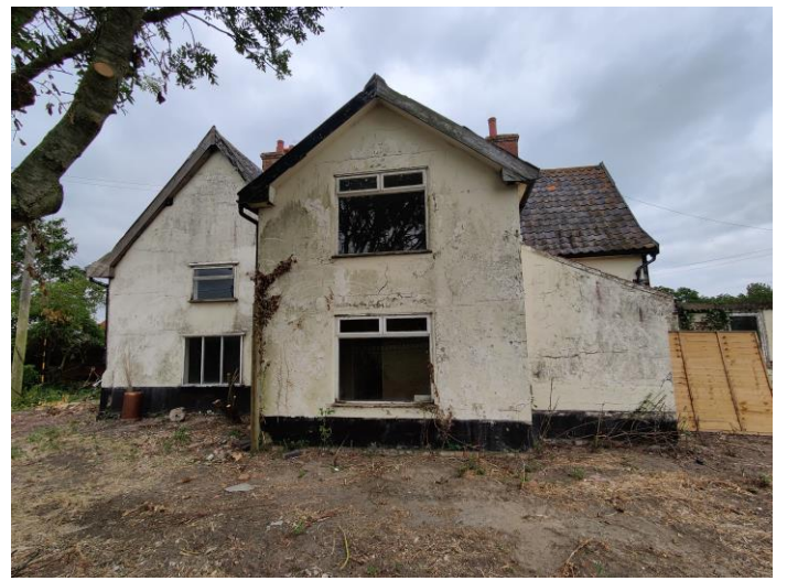
Photo 2 South elevation of buildings B1 (left) and B2 (right)
