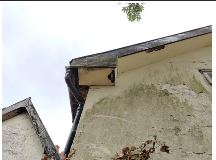
Photo 8 Cavity on soffit box of building B1
