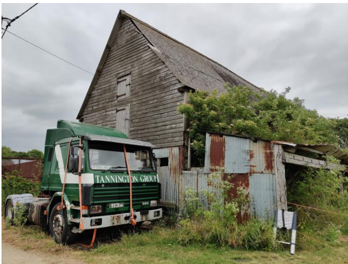
Photo 5 Barn – west and south elevation
