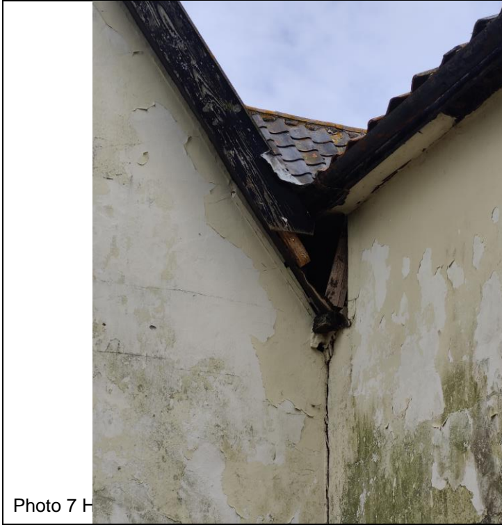
Photo 8 Cavity on soffit box of building B1
