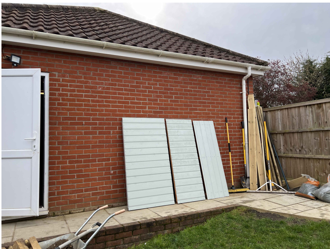
VIEW EAST TOWARD GARAGE WALL
