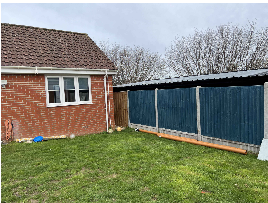
NORTHERN BOUNDARY WITH SHED BEYOND
