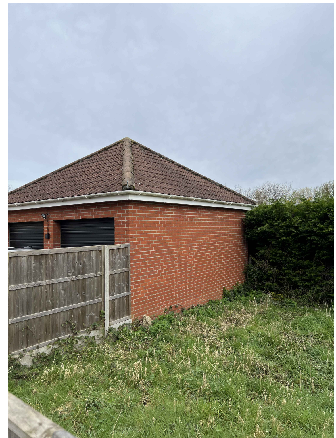
VIEW WEST TOWARD GARAGE
