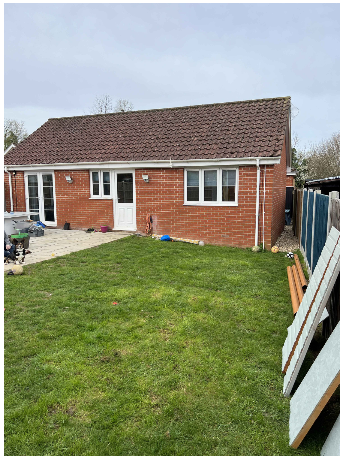
VIEW WEST TOWARD BUNGALOW
