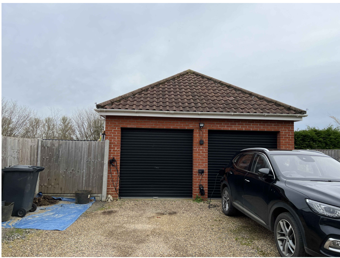
VIEW OF FRONT ELEVATION OF GARAGE
