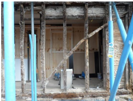
R/H degraded framing to be retained and new frame inserted to support. Red areas marks section of mid rail and base of corner post to be replaced. Remaining mid rail to be retained
