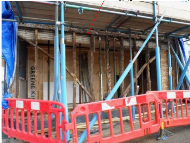
Section of remaining historic timber framing (outline in red above)
