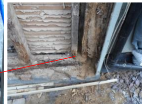
R/H degraded framing to be retained and new frame inserted to support. Red areas marks section of mid rail and base of corner post to be replaced. Remaining mid rail to be retained
