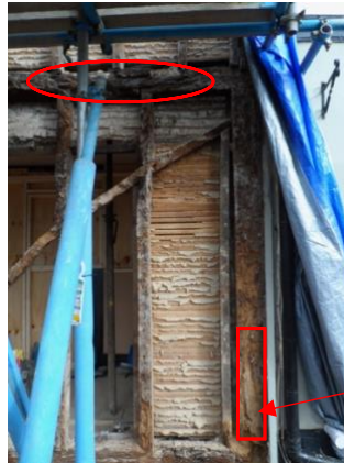
R/H degraded framing to be retained and new frame inserted to support. Red areas marks section of mid rail and base of corner post to be replaced. Remaining mid rail to be retained
