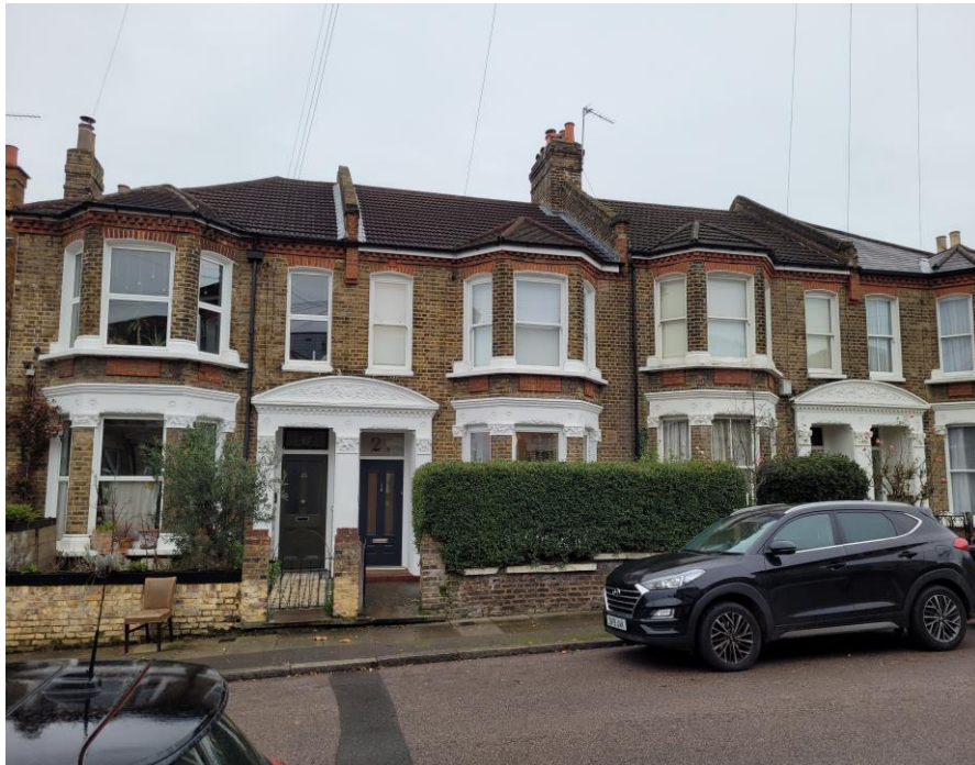
Front elevation of 27 Reservoir Road
