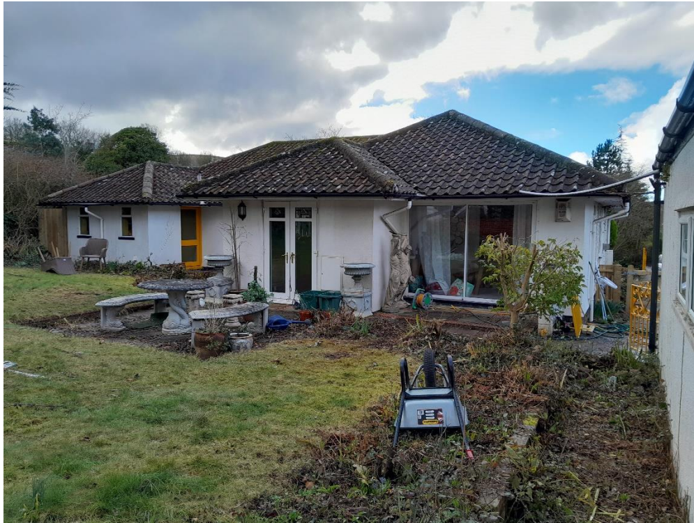
Photo 3. Rear of the dwelling
