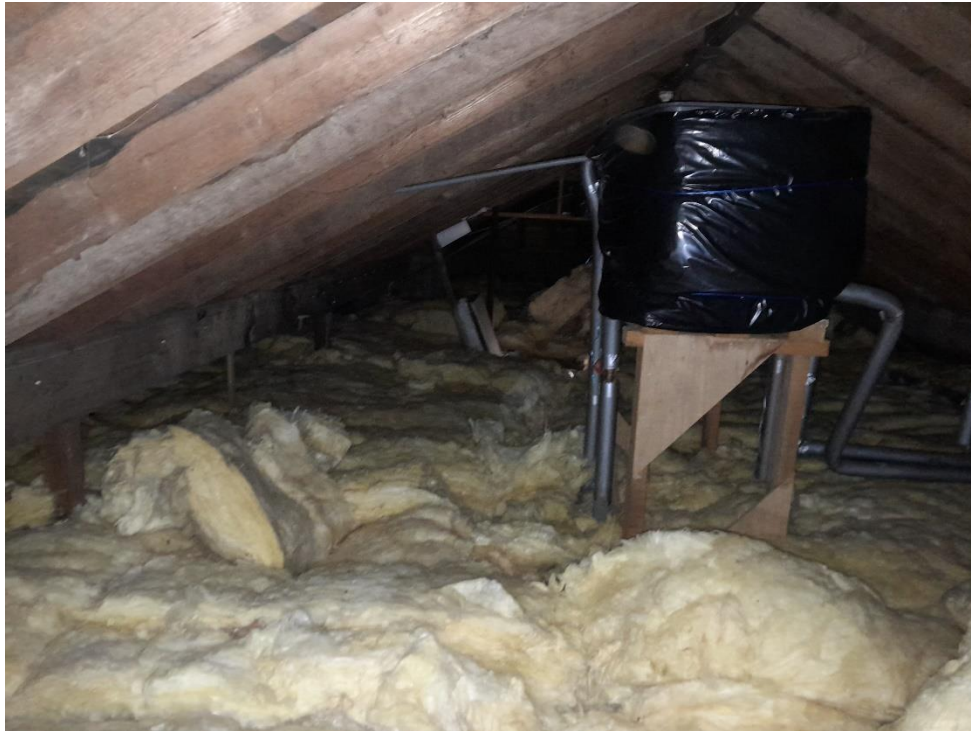
Photo 7. Inside the dwelling loft space.
