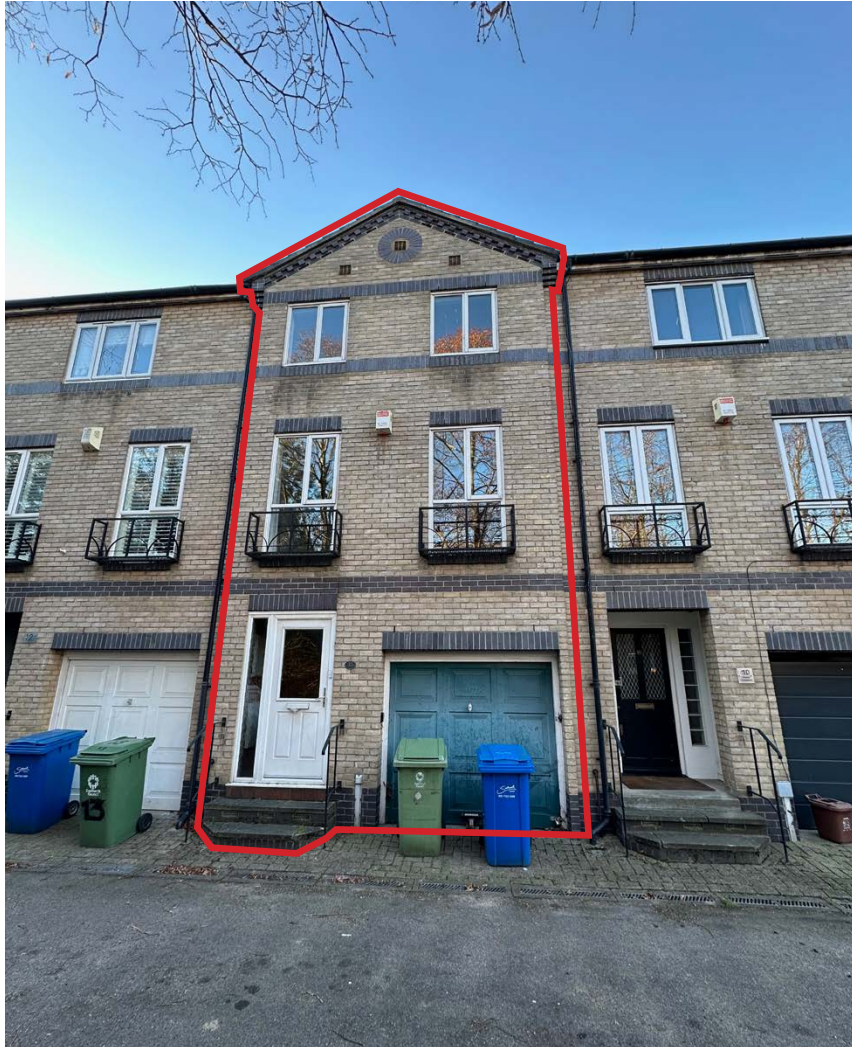
Front elevation. The existing timber framed windows are in poor condition and will be replaced, with white framed double glazed aluminium units. The metal garage door is visually dominant in the elevation and will be replaced with a fixed metal panel with the appearance of a garage door.
