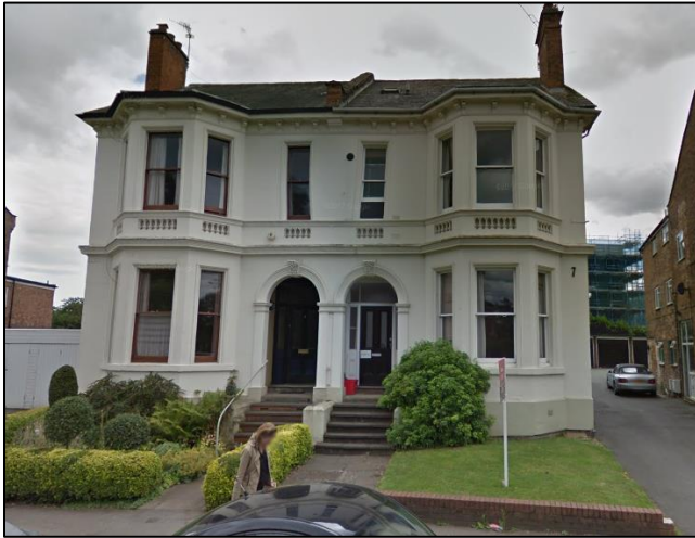
7 Avenue Road ©Google
