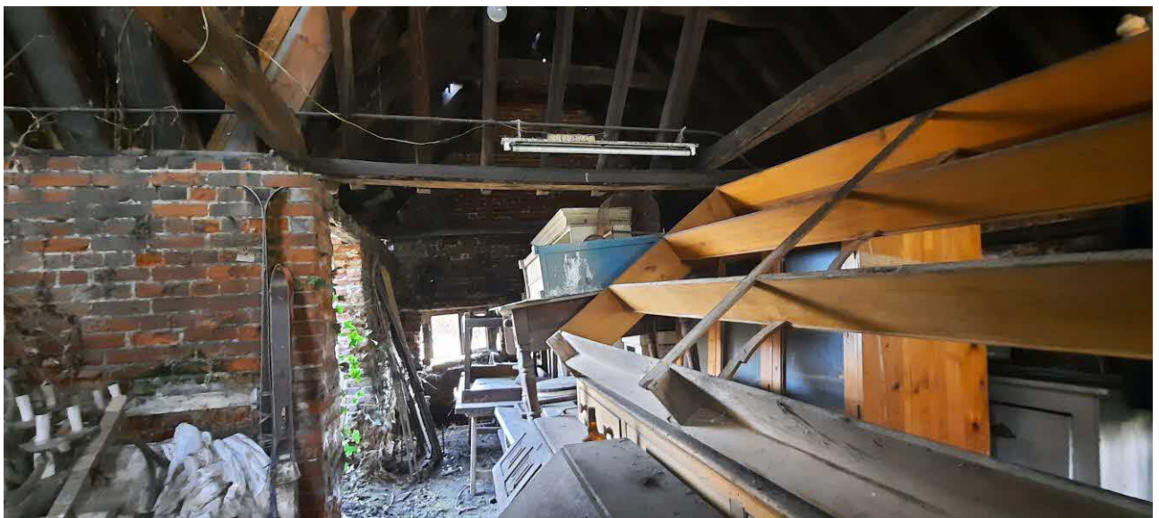
Fig. 8 – view from within The Forge looking towards the rear (and the location of the collapsed lean-to/out-shot). This photograph was taken prior to the purchase of the building and, as is evident, it was used for storage purposes by the previous owners
