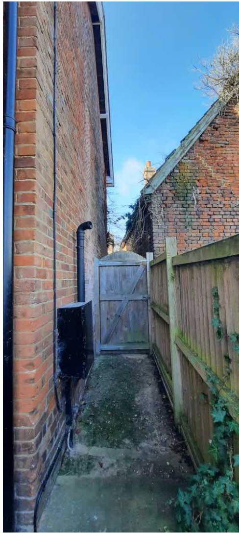
Fig. 7 – view looking west along the side alley to Forge House (north elevation of Forge House and south elevation of The Forge). The proximity of The Forge to Forge House is evident
