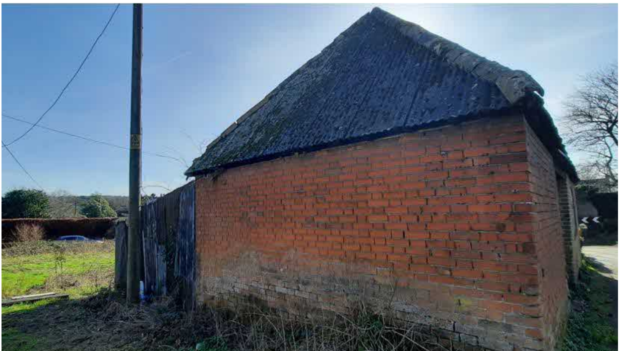
Fig. 3 – the side (north) elevation of The Forge
