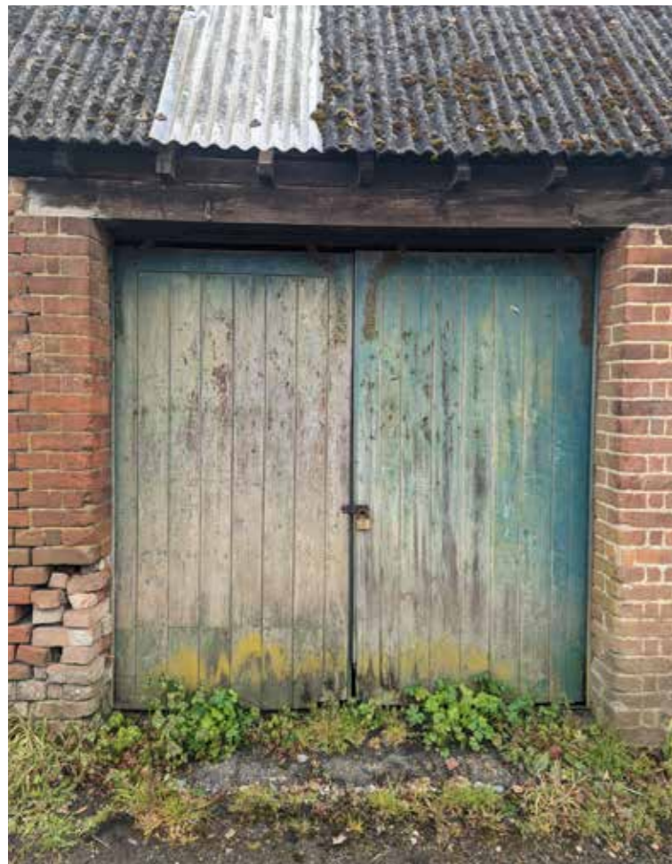
ORIGINAL CART DOORS (GOODNESTONE ROAD)
