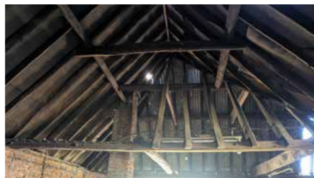
EARLY FORGE ROOF STRUCTURE
