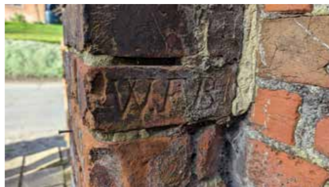
MARKINGS ON BRICK BUTTRESS (INITIALS OF THE LATER FORGE BUILDER?)
