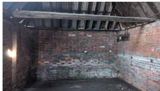
LATER FORGE AND COBBLED FLOOR. NOTE ELECTRICAL DIS' BOARD TO THE TOP RIGHT
