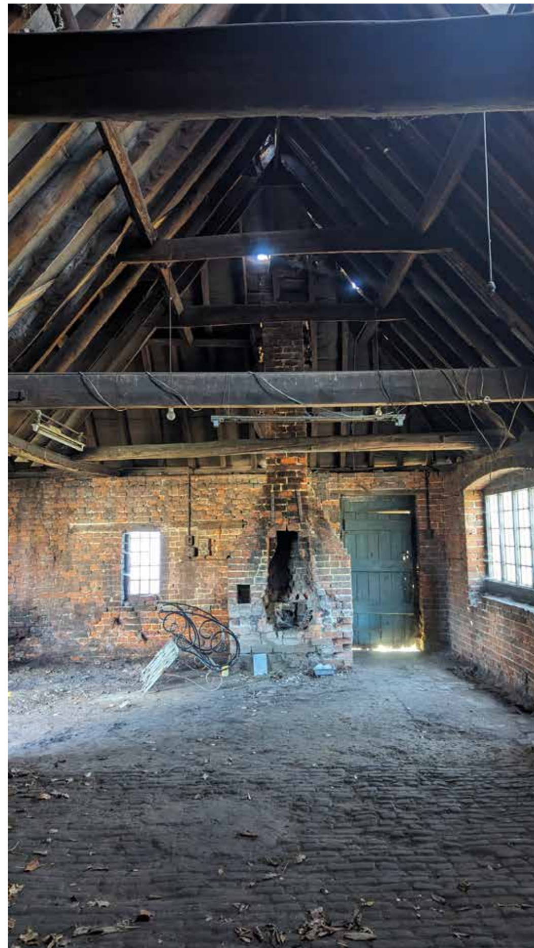
LATER FORGE, COBBLED FLOOR AND (LATER) FURNACE AND CHIMNEY STACK
