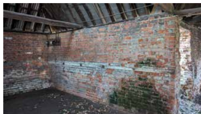
LATER FORGE AND COBBLED FLOOR. NOTE ELECTRICAL DIS' BOARD TO THE TOP RIGHT AND SIDE OPENING, LEADING INTO EARLY FORGE.
