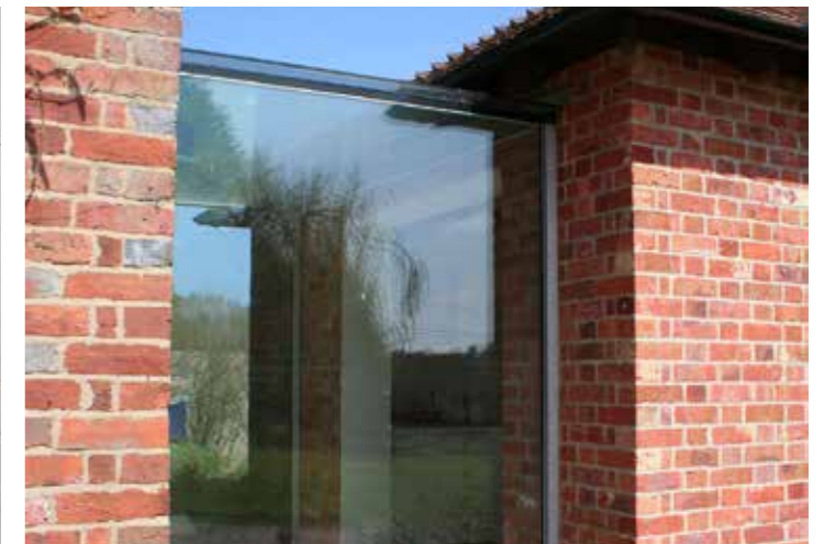
GLASS DOOR ABUTMENT TO OLD BRICK (LIGHT)
