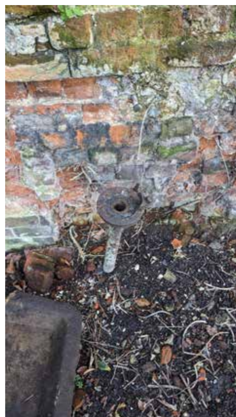
EARLY FORGE WATER SOURCE TO BELOW REAR GABLE (CONNECTED TO WELL)
