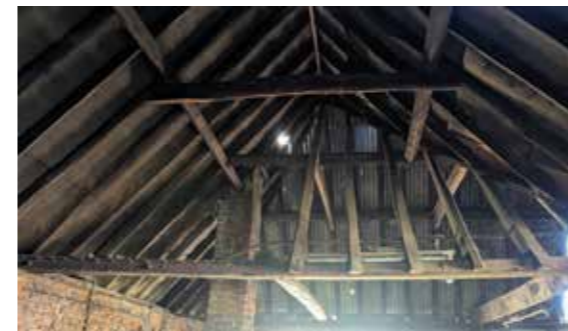
EARLY FORGE ROOF STRUCTURE
