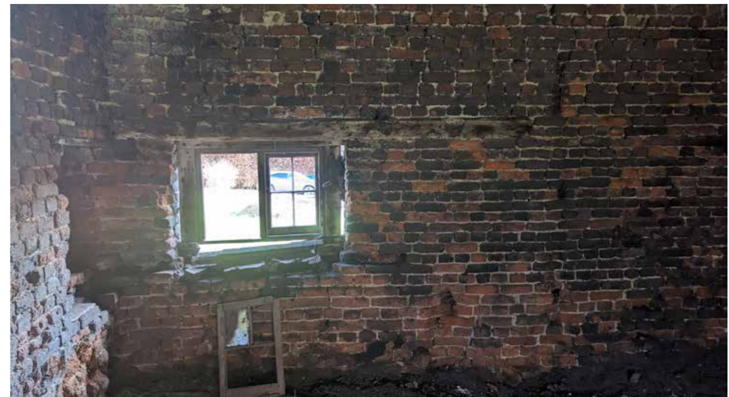
(INTERNAL) EARLY FORGE CASEMENT WINDOW
