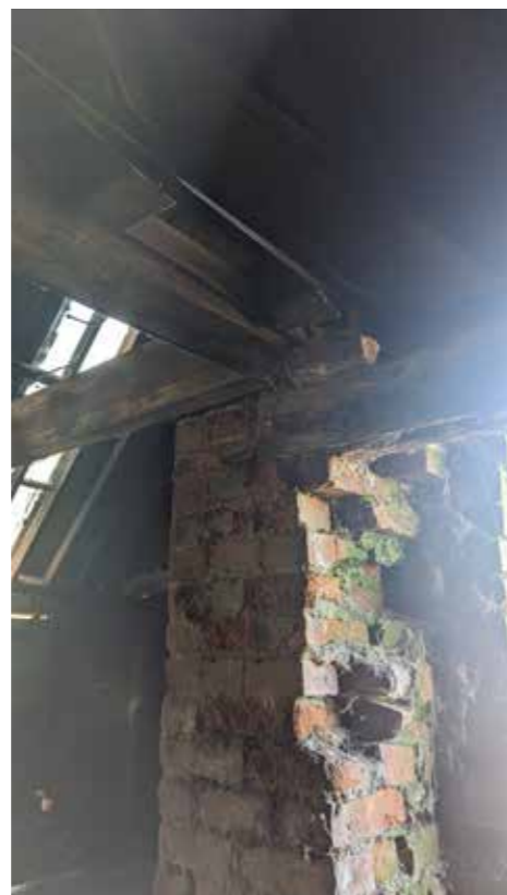
JUNCTION OF EARLY AND LATER FORGE AND SIDE OPENING
