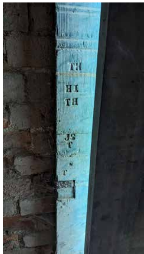
LATER FORGE MARKINGS ON THE FRAME OF THE CART DOORS
