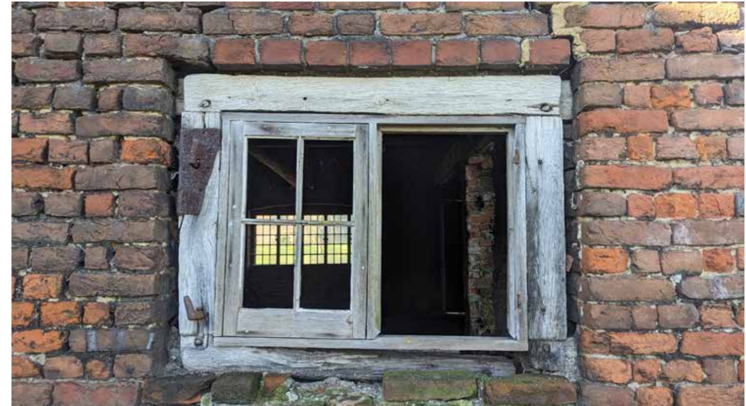
(EXTERNAL) EARLY FORGE CASEMENT WINDOW
