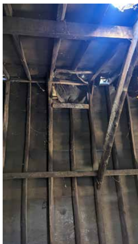
EARLY FORGE'S CHIMNEY ROOF OPENING (REMOVED)
