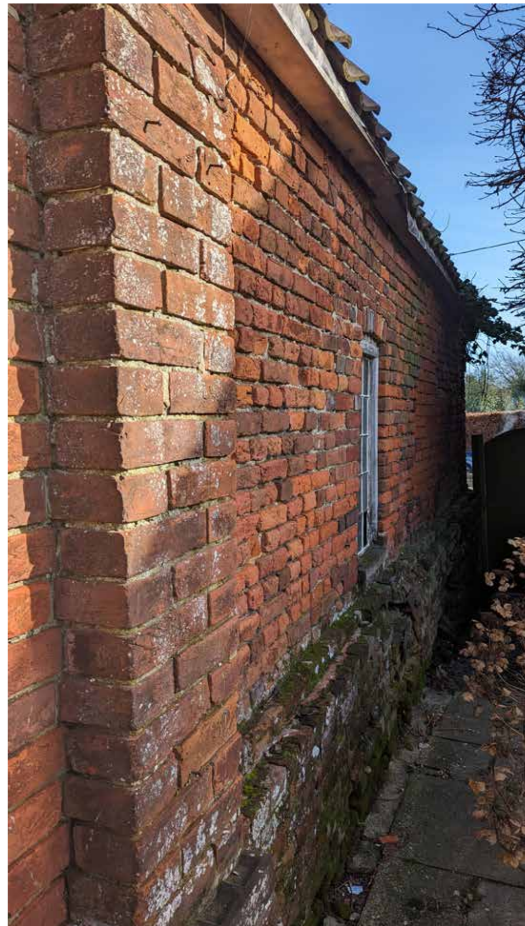
BUTTRESS DEFINING LATER FORGE (FOREGROUND) AND EARLY FORGE (BACKGROUND)
