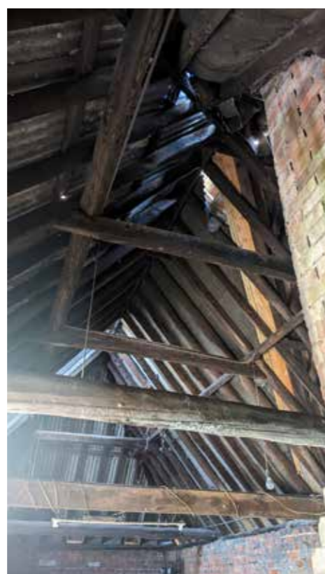
EARLY FORGE ROOF STRUCTURE
