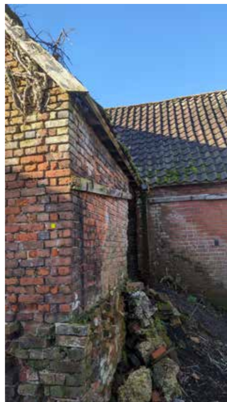
EARLY FORGE AND LATER FORGE IN BACKGROUND, WITH DIRT MOUND.
