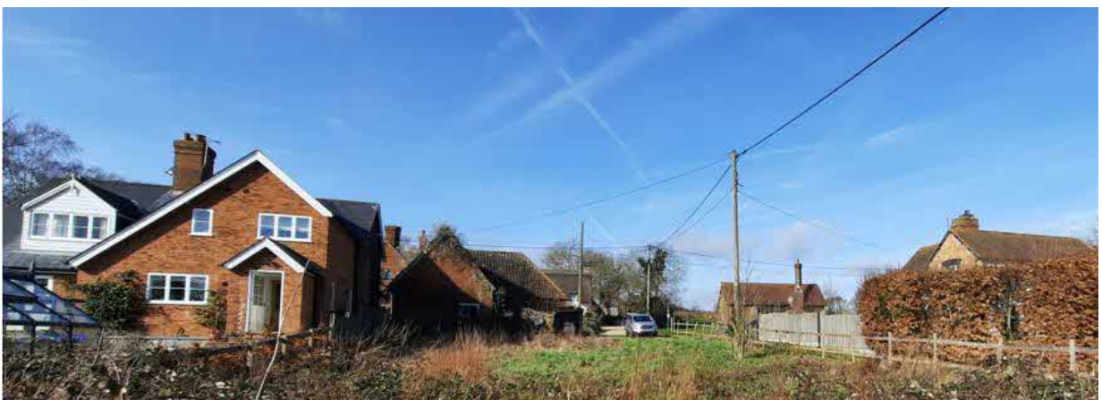
Fig.6 – view looking west to the rear of The Forge (and Forge House) from the car parking area serving Forge House
