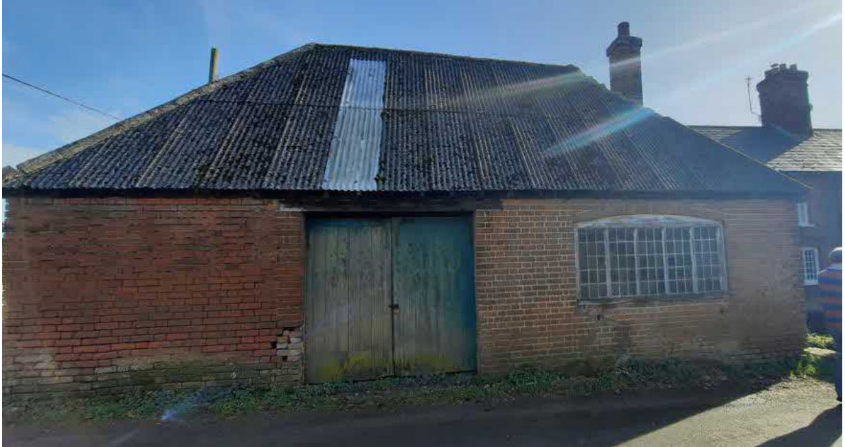
Fig.2 – the front (west) elevation of The Forge
