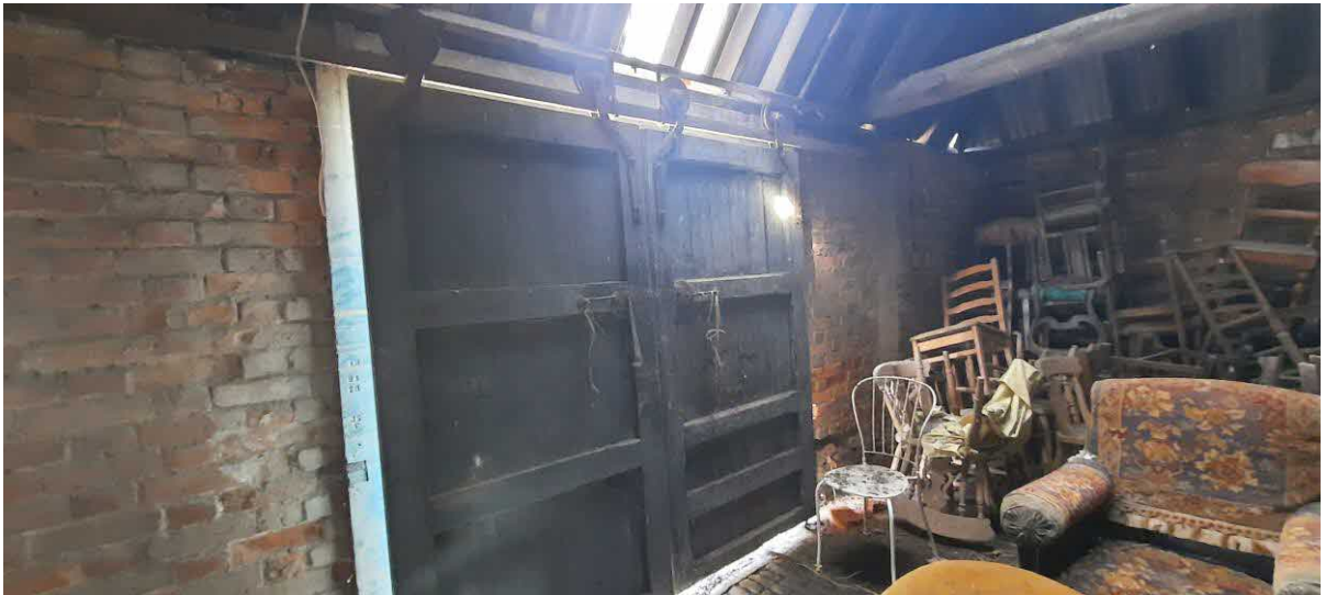
Fig.10 – The Forge interior. View of the front barn/cart-style doors
