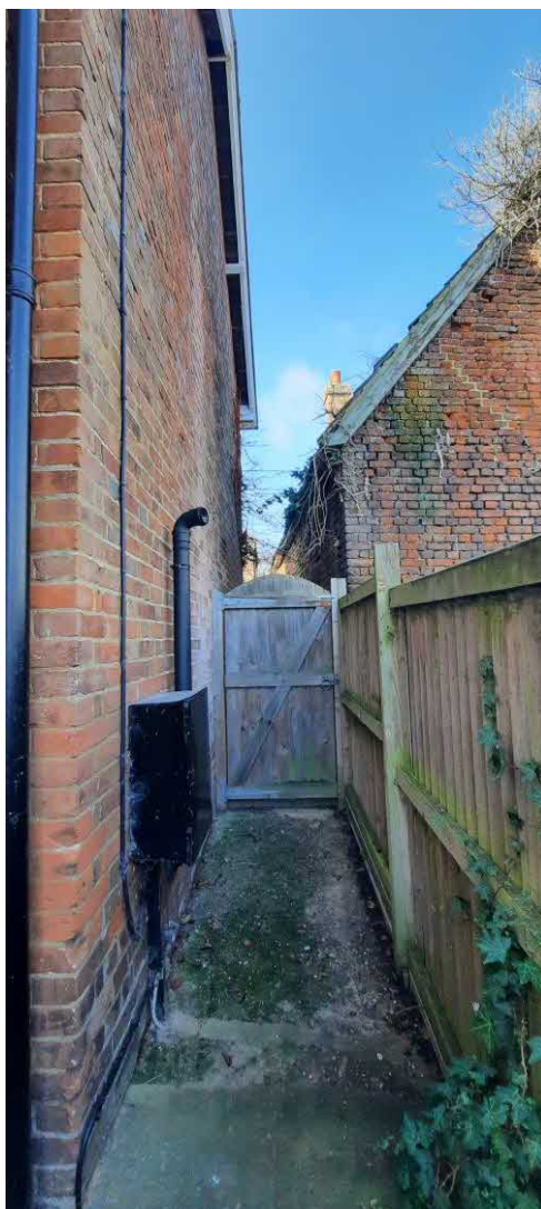
Fig. 7 – view looking west along the side alley to Forge House (north elevation of Forge House and south elevation of The Forge). The proximity of The Forge to Forge House is evident
