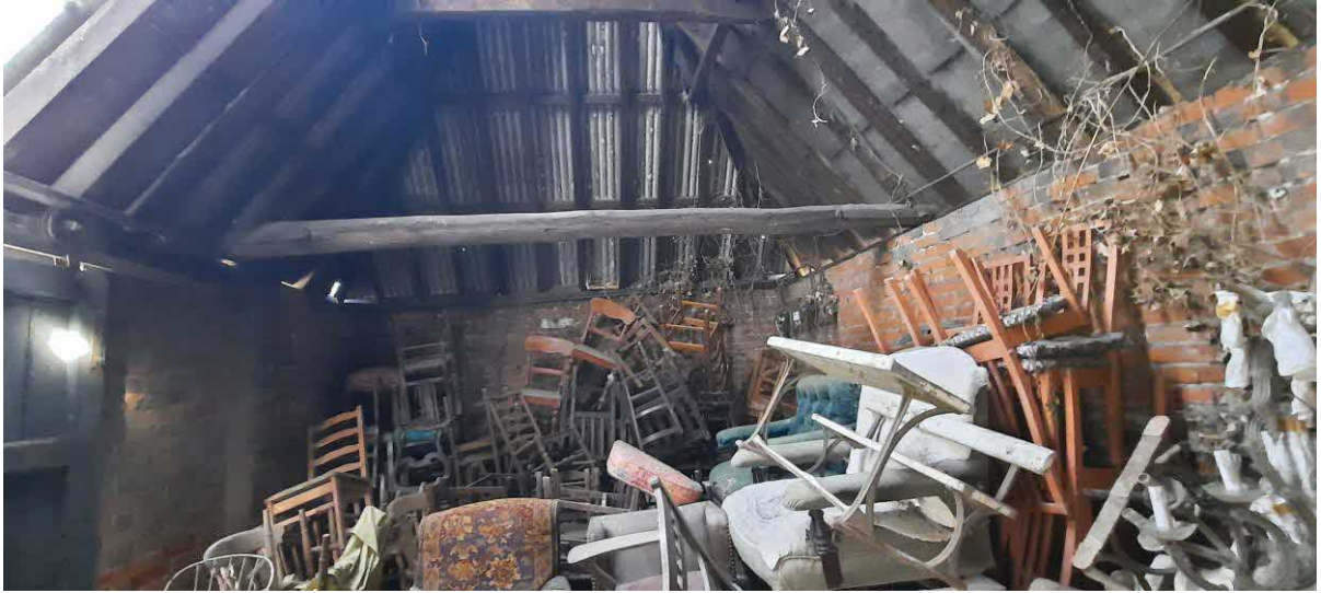
Fig.9 – part of the Forge interior with the front doors evident on the left of the photograph
