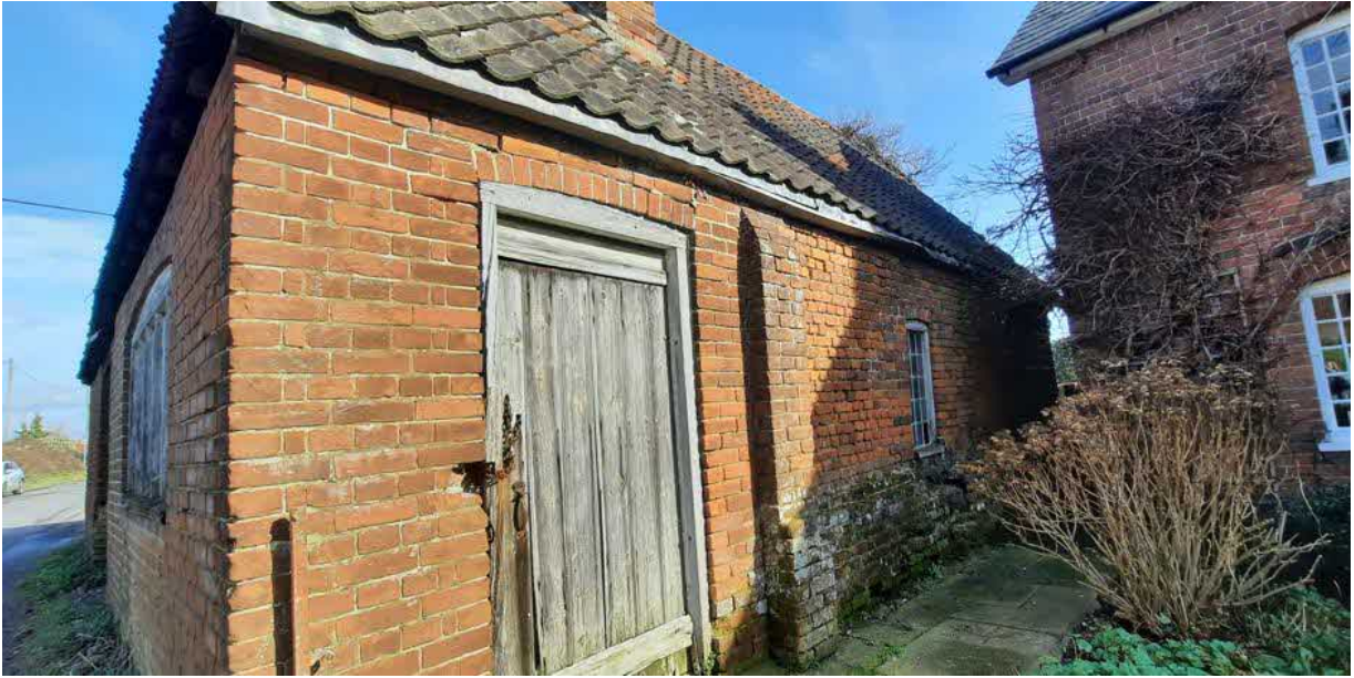
Fig.4 – the side (south) elevation of The Forge closest to Forge House
