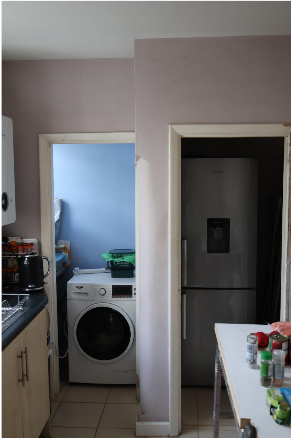
Photograph 4: Interior rear wing (kitchen) number 37 looking south toward the two ancillary spaces. It is proposed to remove the wall and doorcase to the left to incorporate the area containing the washing machine into the kitchen. The partition with the squinch moulding will be retained. Note the door architraves are modern as is the floor and the wall surfaces.
