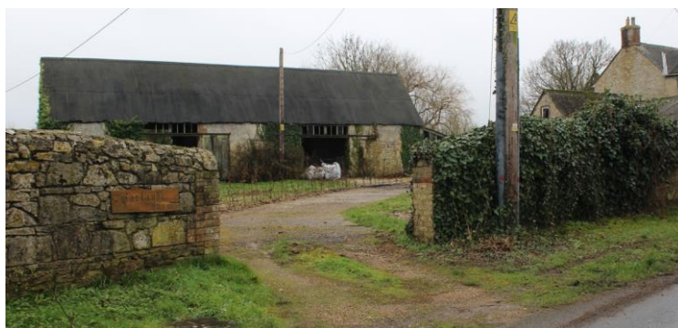
Access to be widened
