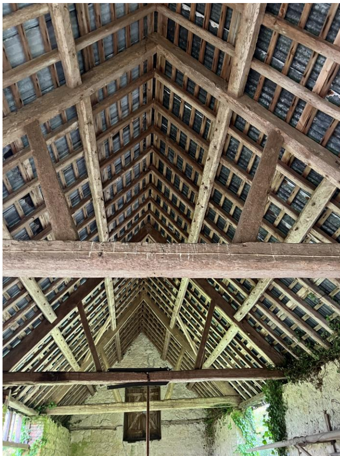
Photo 4 The interior of the roof of the barn
