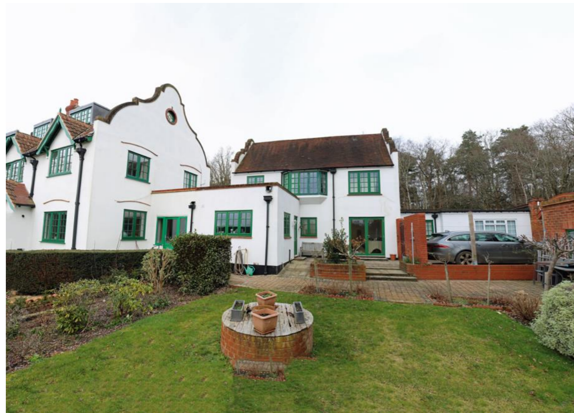
View of South Elevation of Heather Hills Cottage
