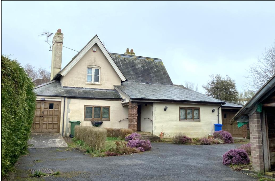
View of existing house
