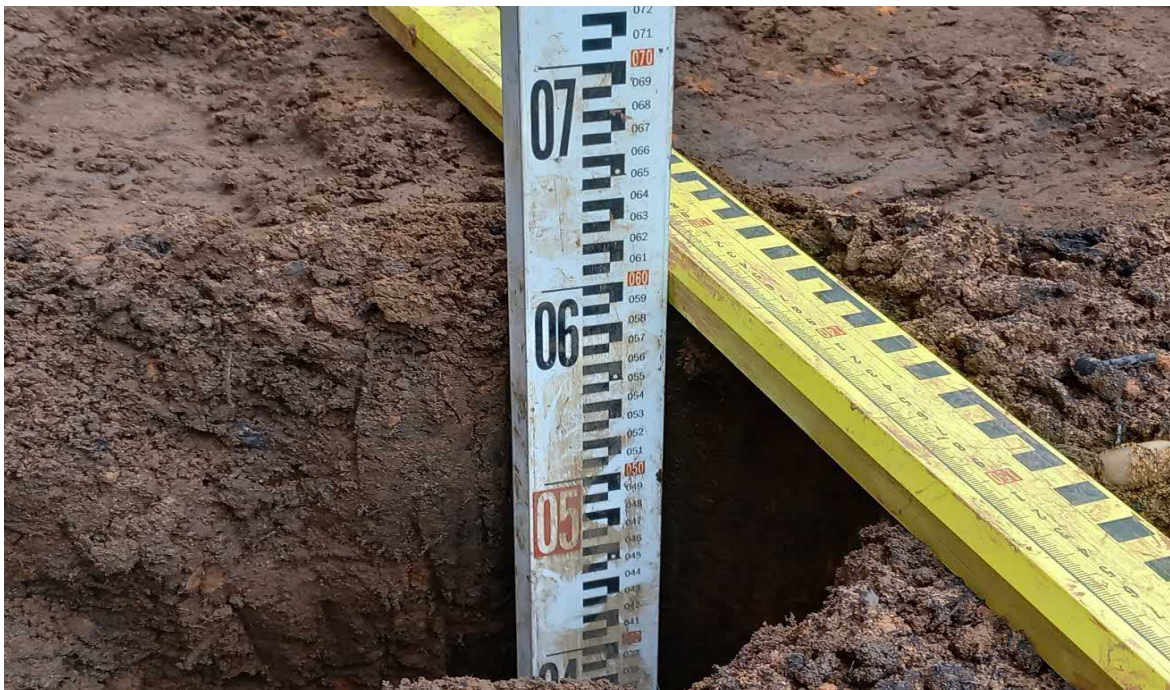
Photo 8: Internal view of S3 excavation.
