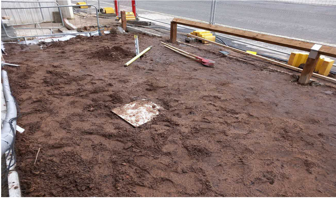
Photo 13: Overview of S5.
