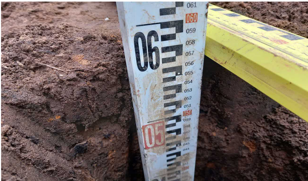
Photo 10: Internal view of S4 excavation.
