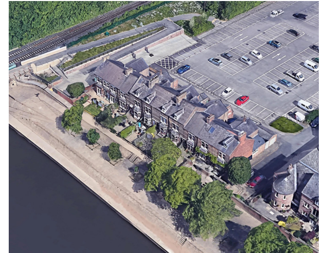
Google earth view of the site
