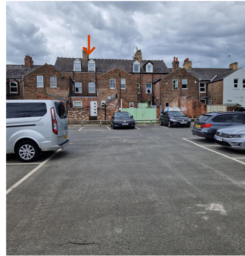
Rear elevation viewed from Marygate car park
