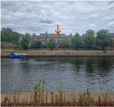
Front elevation viewed from the opposite side of River Ouse
