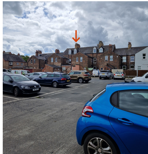
Rear elevation from Marygate car park
