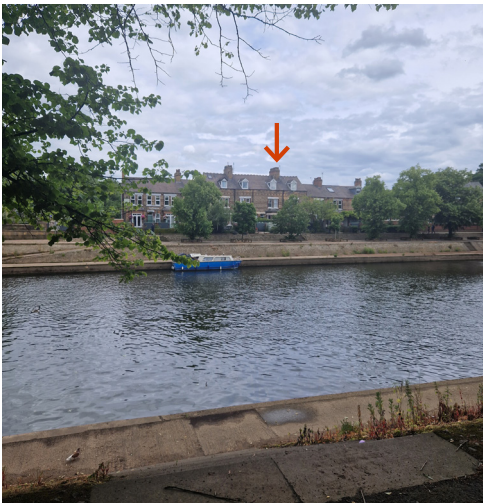
Front elevation viewed from the opposite side of River Ouse
