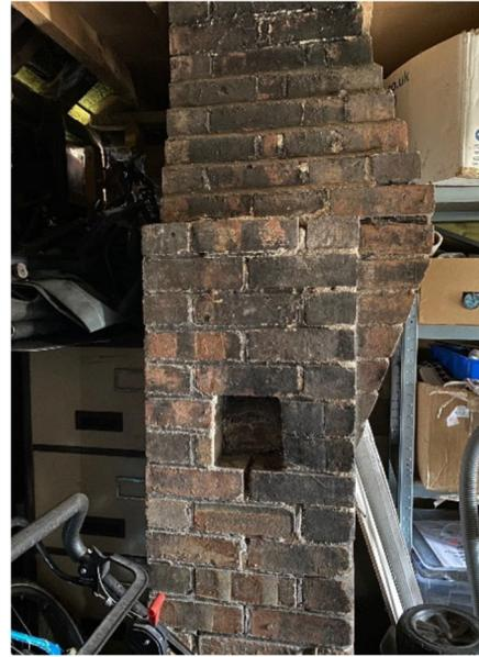
There is an enclosed shed portion on the left side, this houses a chimney which has been removed at an unknown time down to eaves level. It is believed that this is the remains of the original forge chimney.
