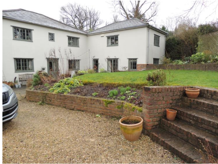
Photo 12: Maintained garden and The Old Forge to the south
