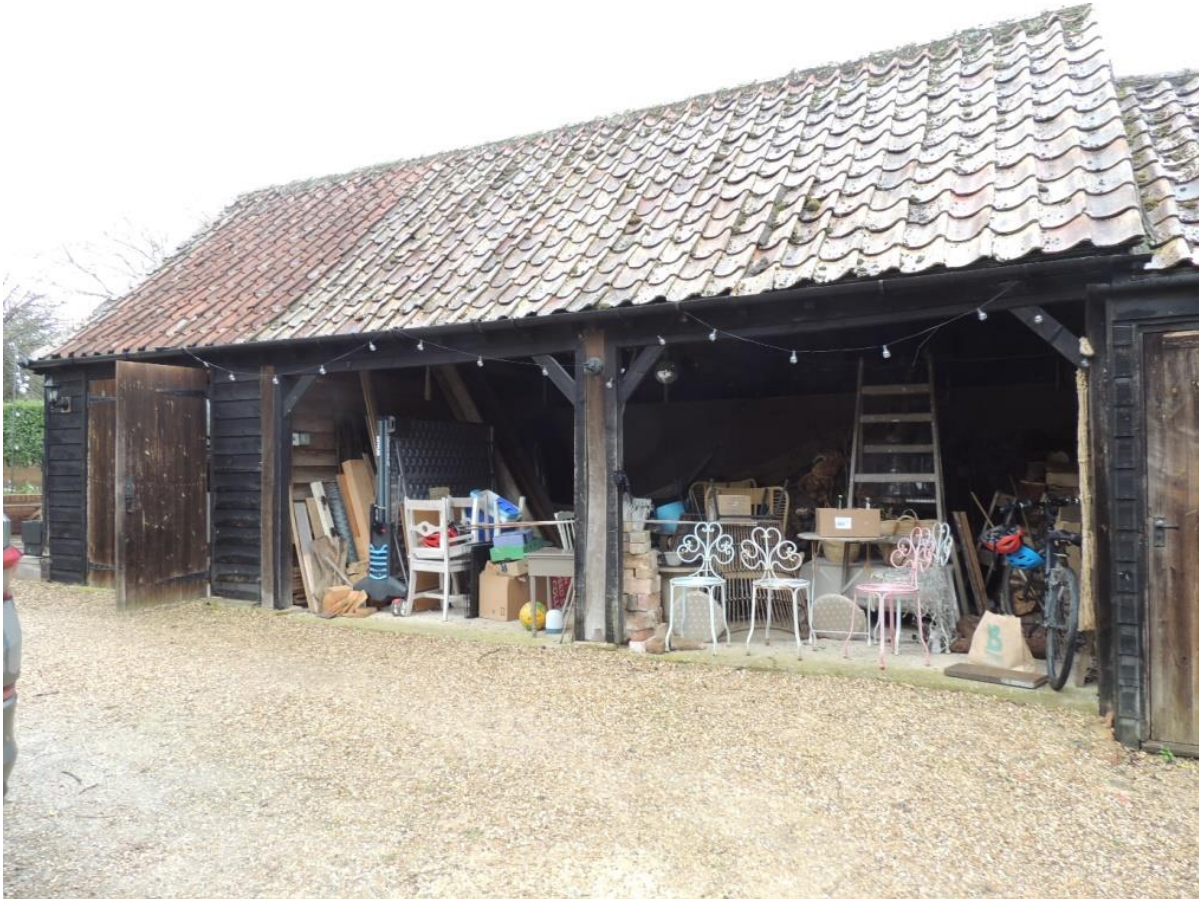
Photo 1: Southern elevation. Note tight seal to roof tiles
