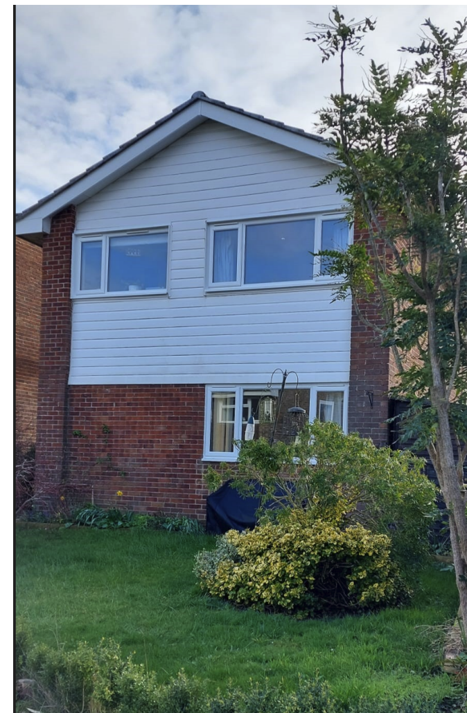
EXISTING FRONT ELEVATION VIEWED FROM FINCH ROAD
