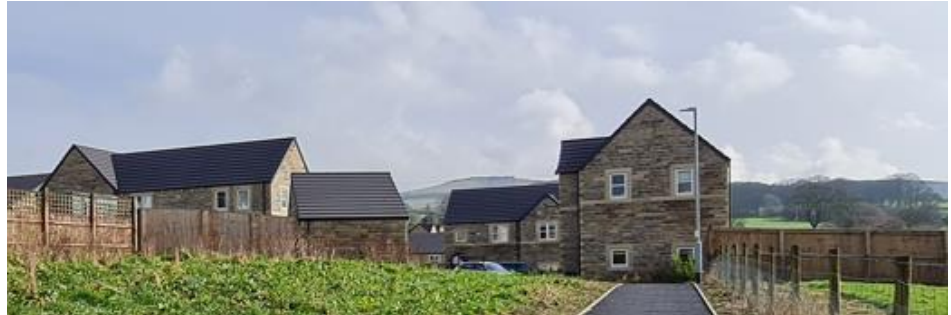
Newly constructed dwellings to the east of the site.
