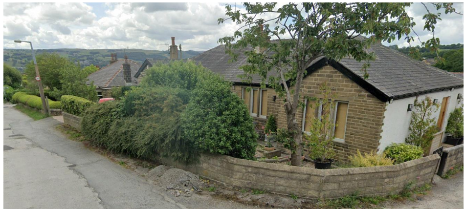
Bungalows opposite the site.
