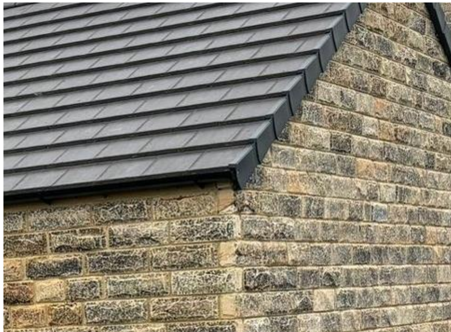
Photograph of the proposed wall and roof materials. Photograph is of the existing garage adjacent to the eastern boundary of the site.
